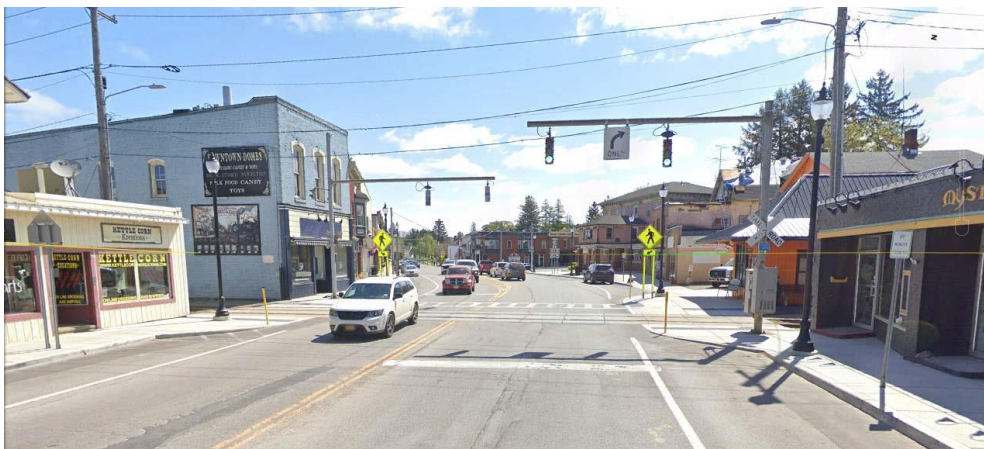
Arcade, NY downtown crossing of Arcade & Attica Railroad with pedestrian crossing; passive rail crossbucks with active traffic signals protecting both pedestrian and rail track crossing. Railroad equipment action triggers stoplight circuit.
