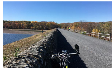
Ashokan rail-trail, Ulster Co. NY. Note width, extensive guard rail system for higher speed
