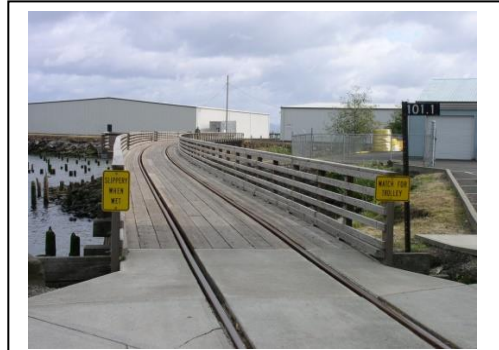
Astoria, OR trail with planked-over rail bridges for dual use.
