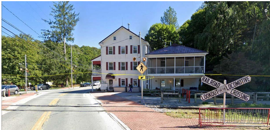
Railroad, PA Northern Central Railroad / York County Rail Trail crossing with parallel trail and track use – passive crossbucks and active flasher for pedestrian traffic. All crossings on this project have pedestrian signage and/or flashers.
