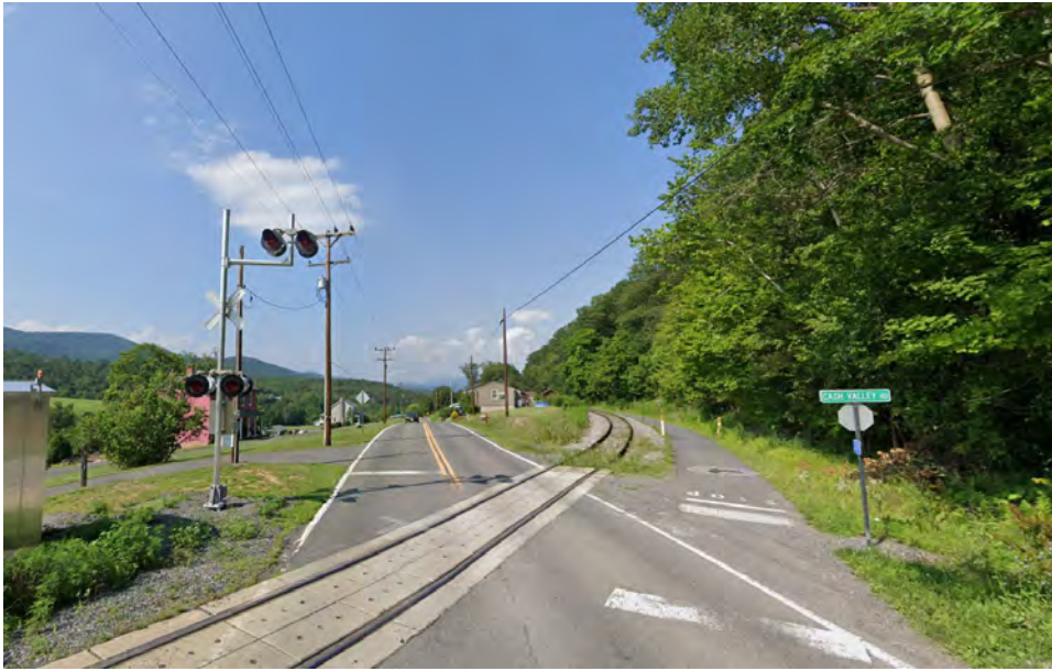
Figure 18: Rail within 6' of edge of trail at Helmstetter's Curve west of Cumberland, MD.
