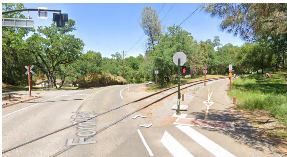
Figure 3: El Dorado Rail Trail crossing Forni Rd in Placerville, CA with reduced separation between the inactive rail line and the paved, shared use, two-way trail.
