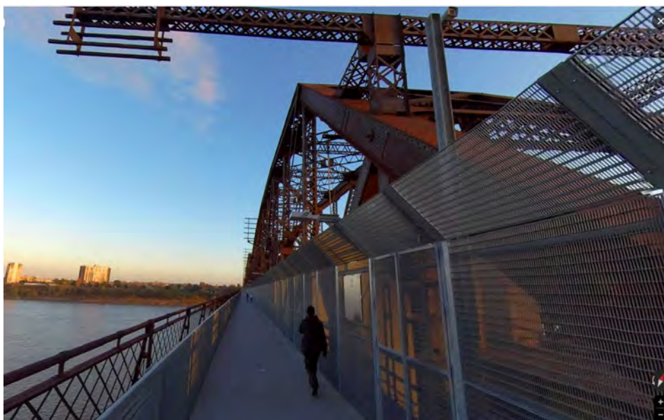
Figure 2: Shared use path attached to the side of the Harahan Rail Bridge across the Mississippi River.
