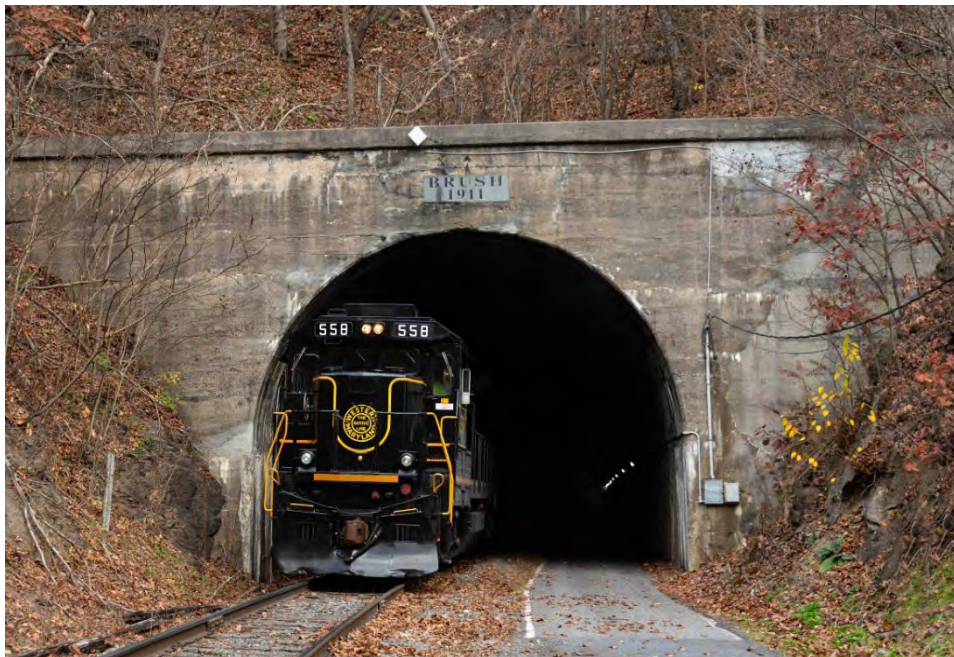
Figure 17: The entrance to the Brush Tunnel, showing less than 6' separation between rail and trail and the scale of the excursion train. Photo provided by wmsr.com.
