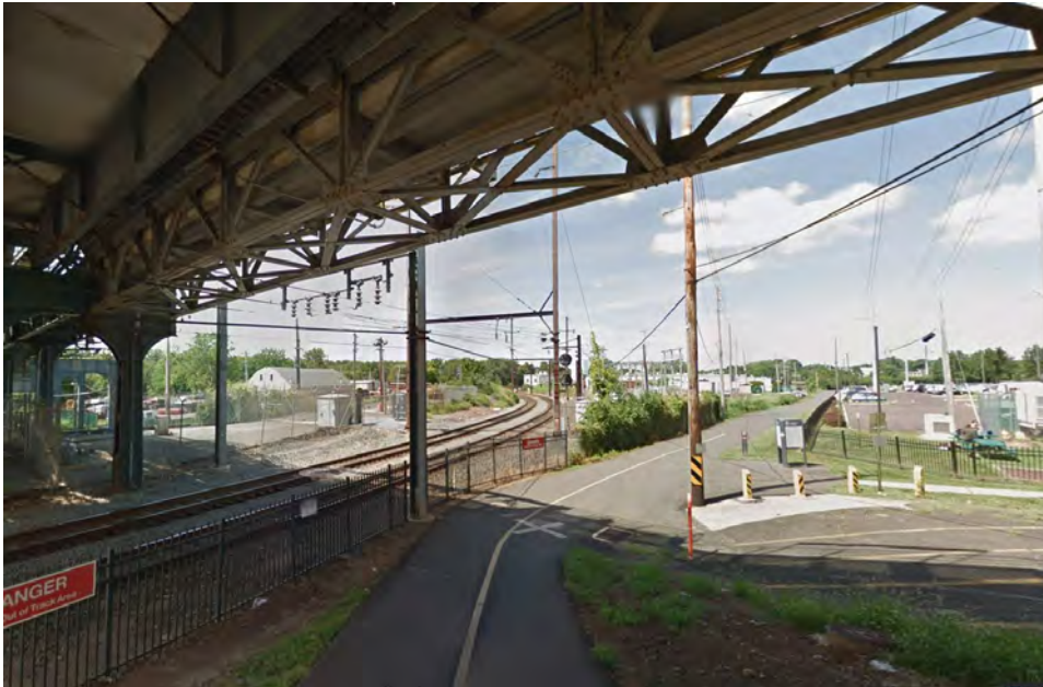
Figure 20: Schuylkill River Trail at Norristown Transportation Center showing brief separation of less than 11' under structure for the SEPTA R100 High Speed Line.
