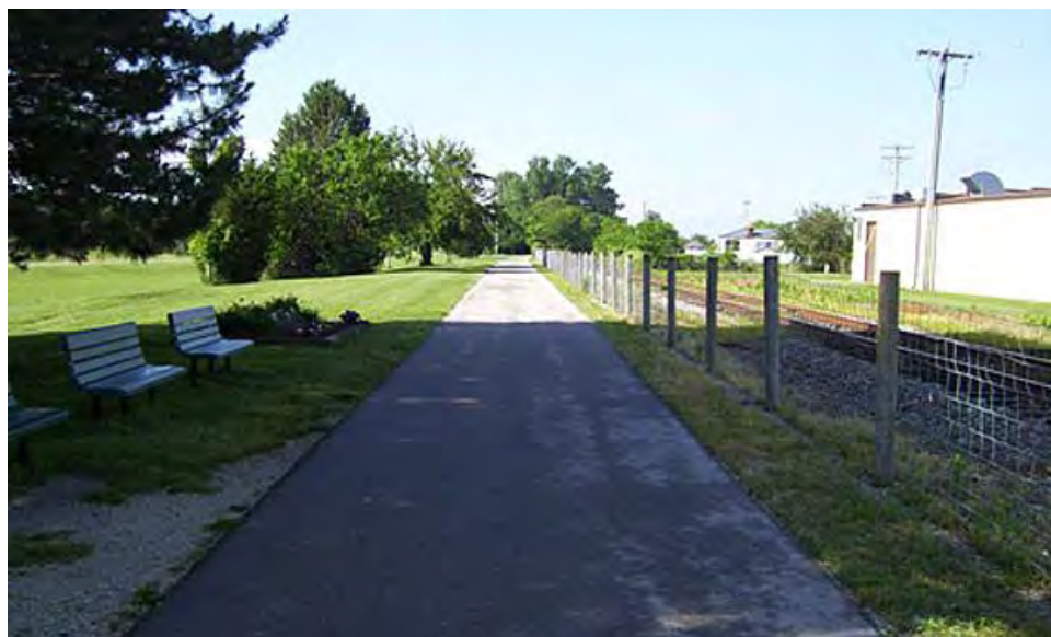
Figure 13: Celina Coldwater Bikeway separated from rail by 10'-12' and a fence. Picture provided by TrailLink.com.
