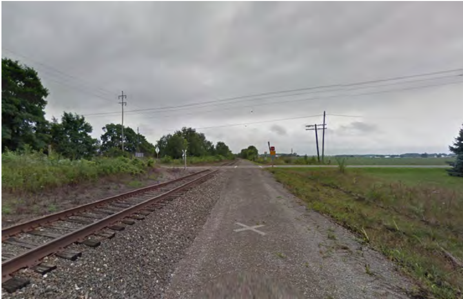
Figure 14: Simon Kenton Trail showing less than 10' separation between rail and trail.
