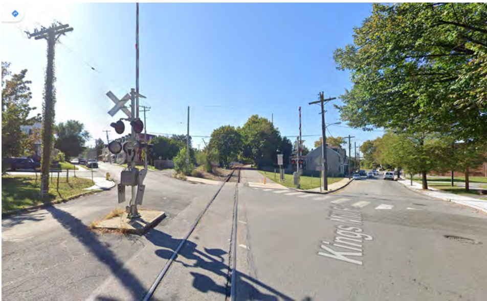
Figure 22: Heritage Rail Trail County Park in York, PA, showing less than 4' separation between the railway and the paved shared use path. Railway is inactive in this section.
