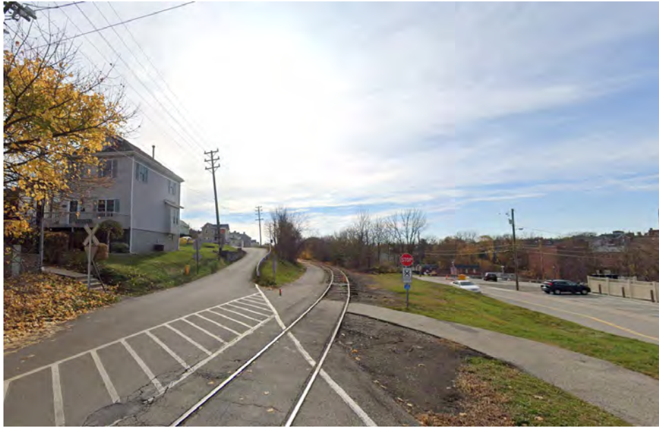
Figure 19: Five Star Rail-with-Trail in Greensburg, PA, showing less than 4' separation between rail and trail.
