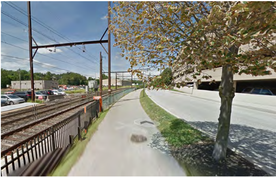
Figure 21: Schuylkill River Trail near the Conshohocken Commuter Rail Station, showing less than 11' separation between the railway and the trail with fencing.
