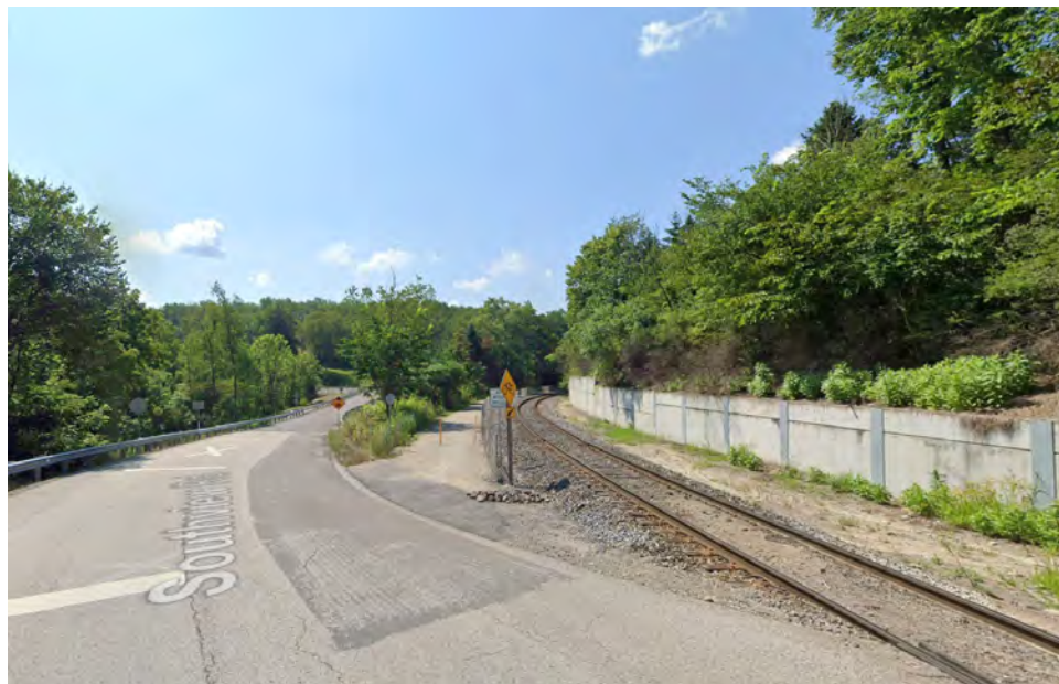
Figure 25: Grade crossing at Southview Rd near McDonald, PA, showing less than 11' separation between Montour Trail and rail.
