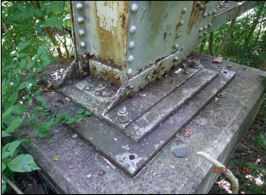
Photo 5: Typical Steel Bent Tower Bearing and Pedestal
