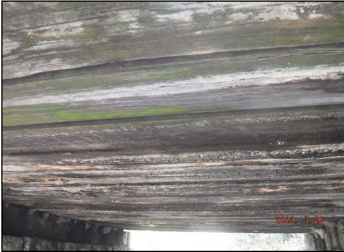
Photo 3: Typical Timber Slab
