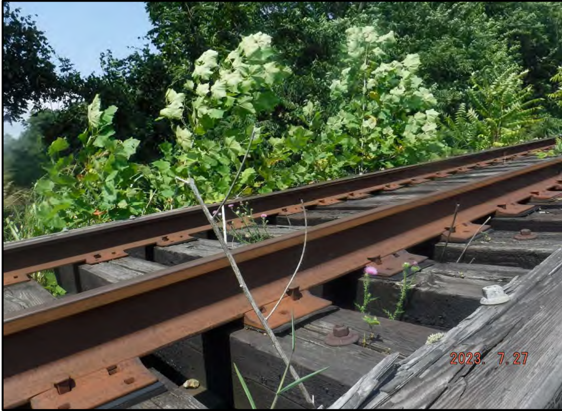
Photo 1: General Condition of Timber Tie Deck
