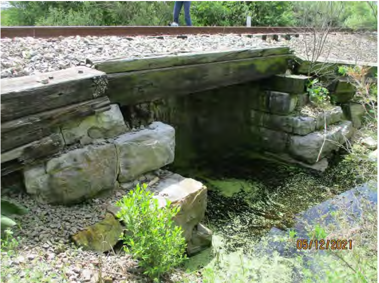
Asset 8763 over Unnamed Drainage Crossing N 38° 43' 39.38", W 78° 39' 39.25" Single Barrel Culvert, 15'-0"
