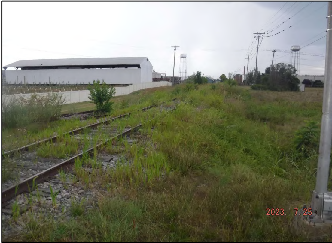
Photo 1: Track on Bridge (From Crossing to the West)
