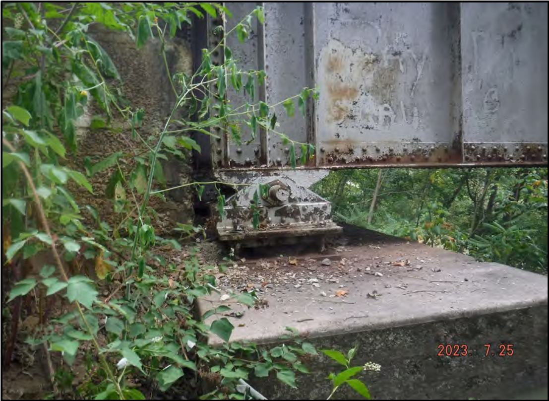
Photo 4: Typical Bearing and West Abutment Bridge Seat (From South)
