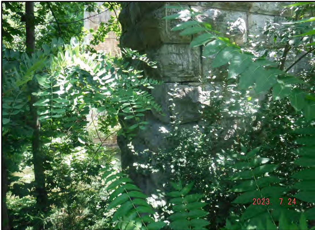
Photo 4: Typical Stone Masonry Portion of Pier
