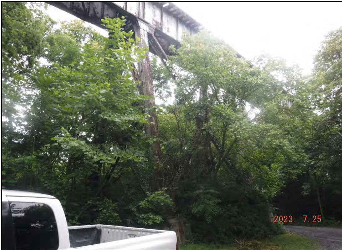
Photo 8: Typical Steel Bent Tower
