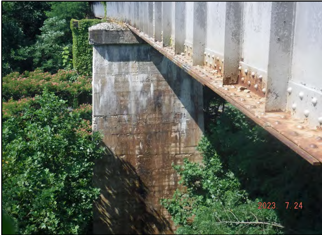
Photo 3: Typical Reinforced Concrete Portion of Pier
