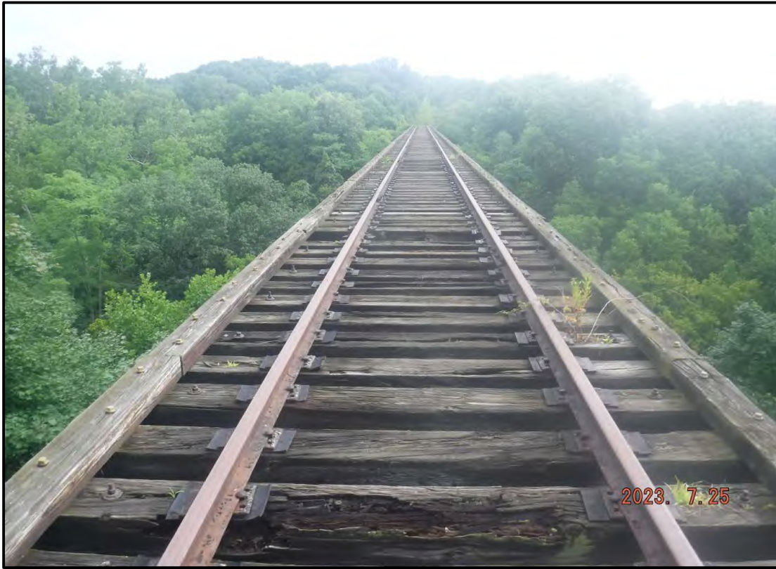
Photo 1: General Condition of Timber Tie Deck
