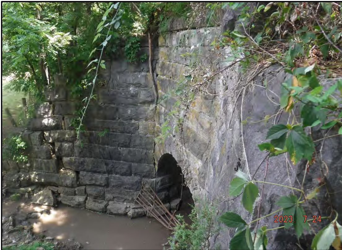
Photo 4: North End of Structure (From NW Wing)
