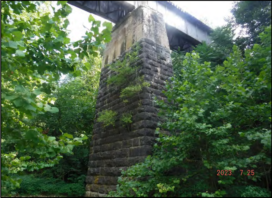
Photo 3: Typical Pier (East Side of Pier 2 Shown)
