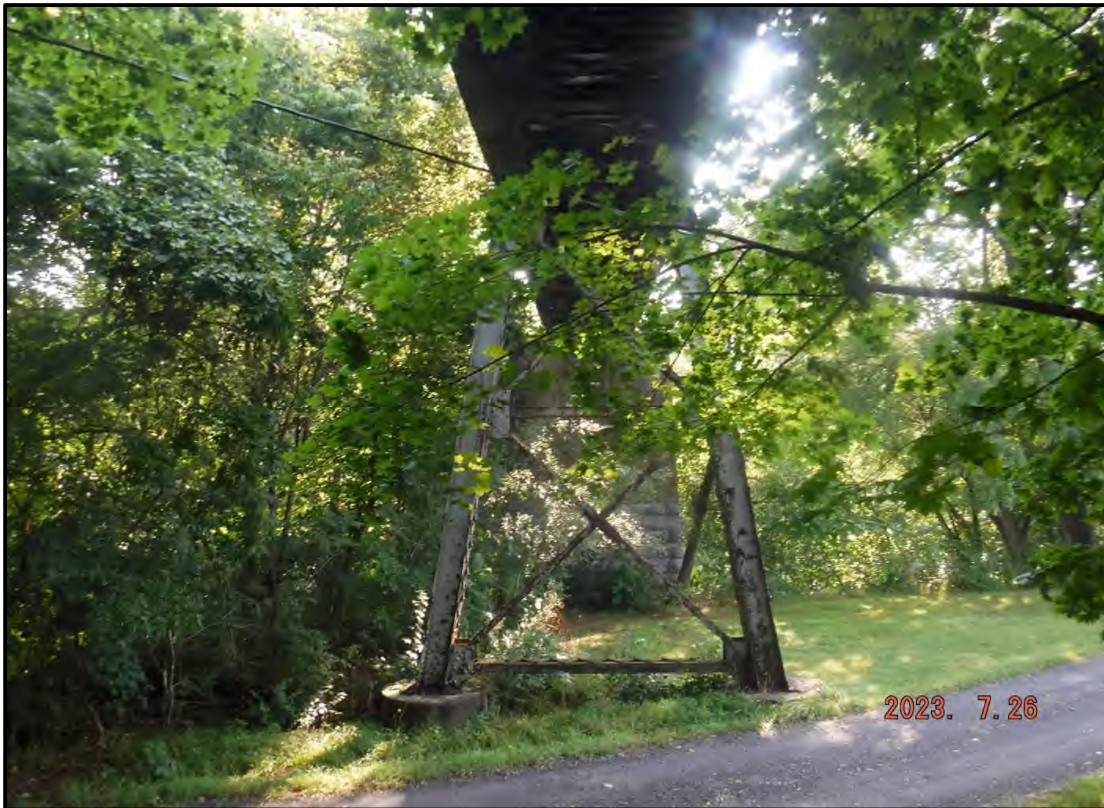
Photo 4: Typical Steel Bent (West Side of Bent 2 Shown)
