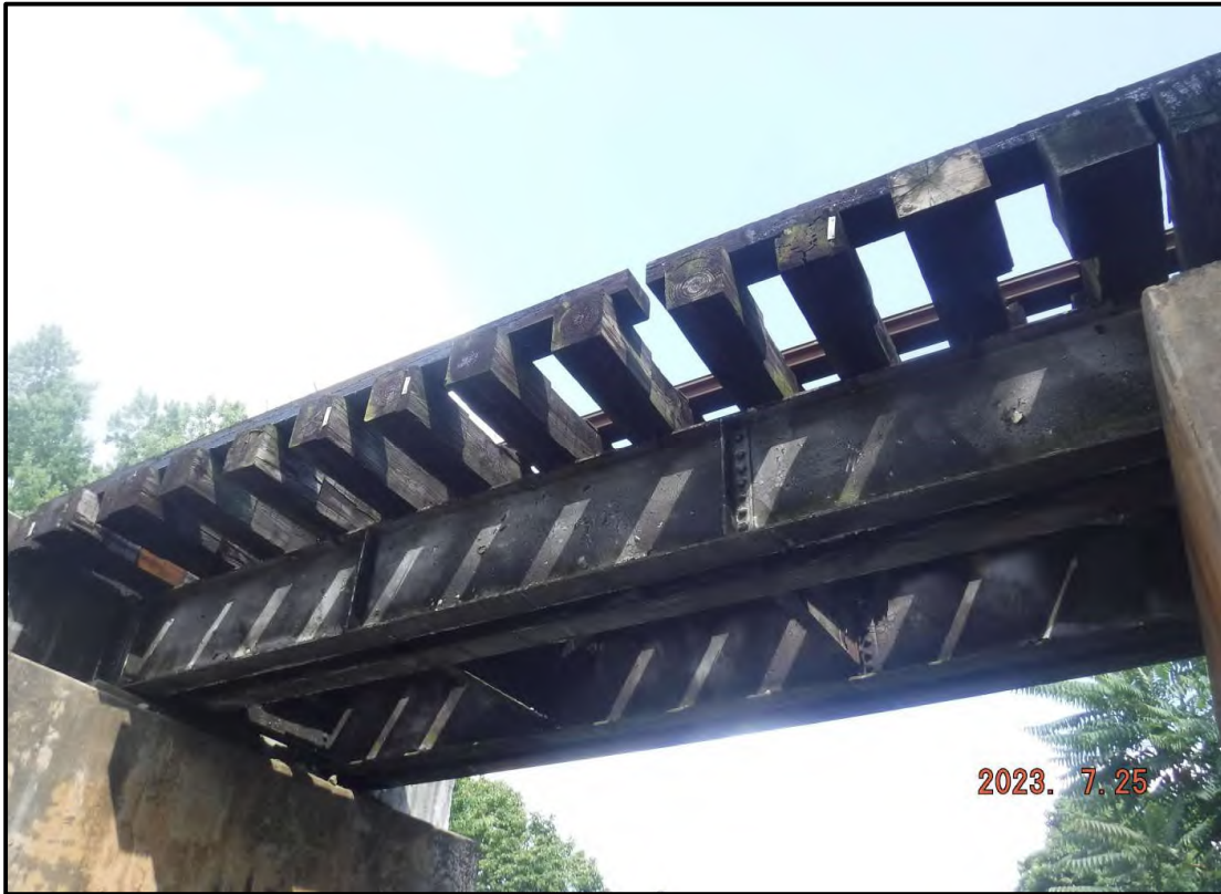
Photo 1: North Elevation of Girders
