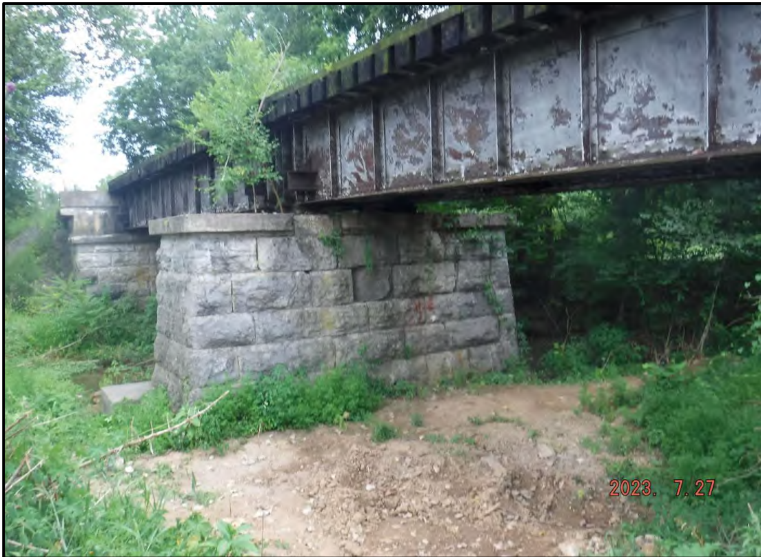
Photo 6: West Side of Pier
