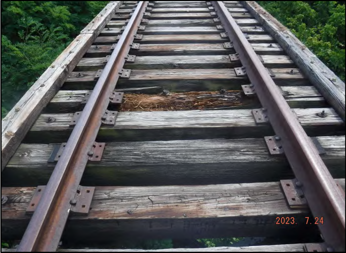
Photo 1: General Condition of Timber Tie Deck
