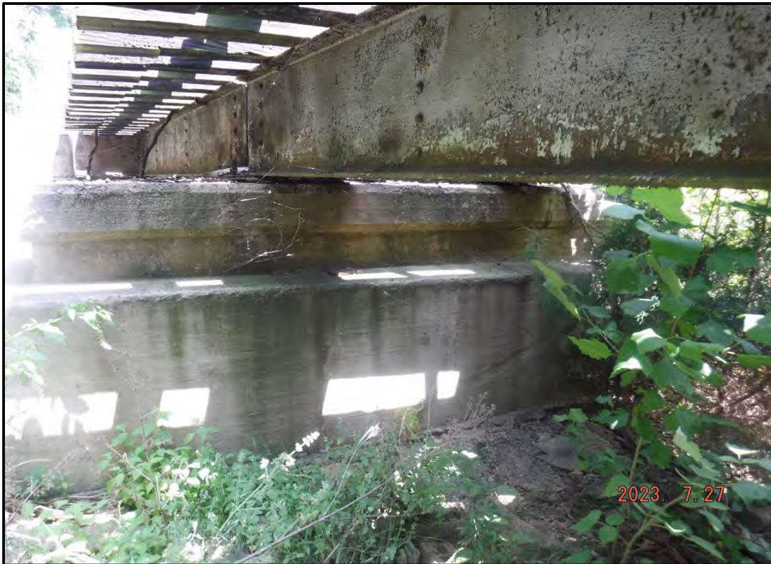
Photo 4: West Side of Pier
