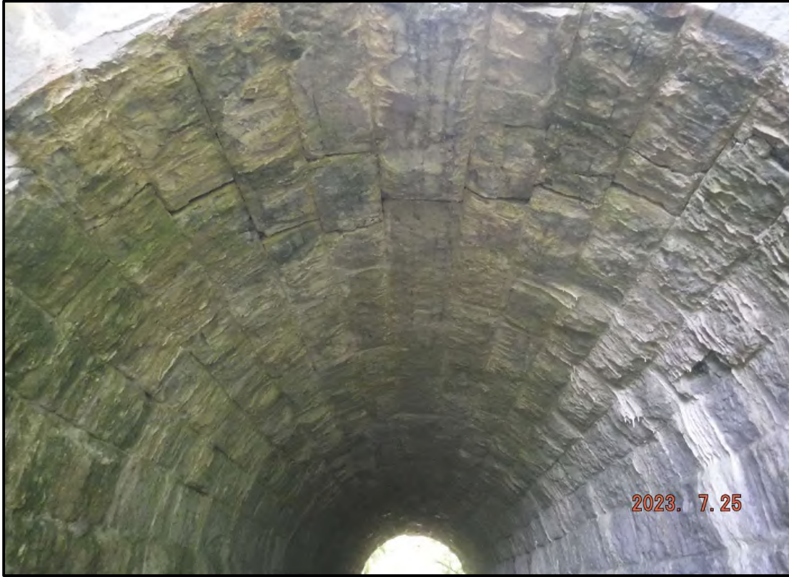
Photo 3: Arch Barrel (From North)
