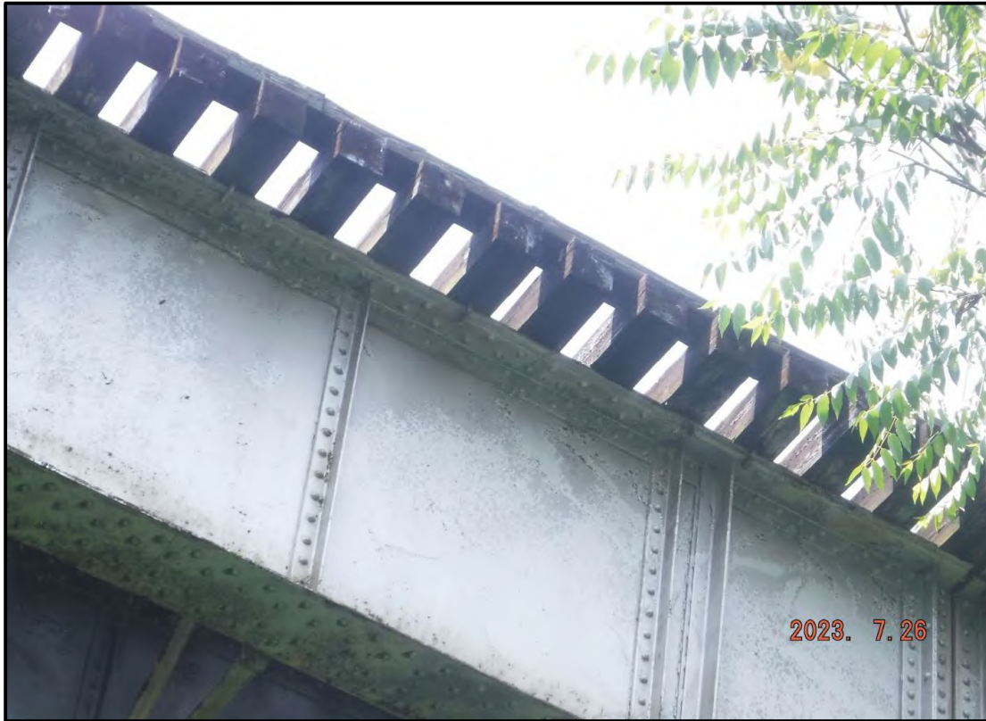
Photo 1: General Condition of Timber Tie Deck
