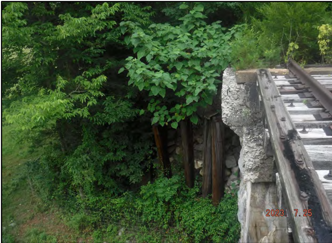
Photo 4: Typical Wingwall (NE Wing Shown)
