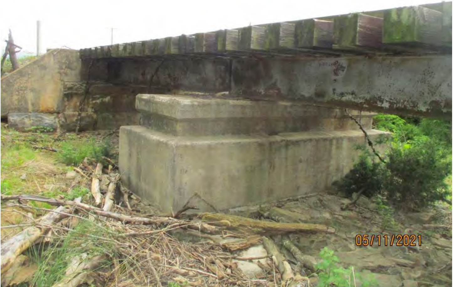
Asset 9435 over Unnamed Drainage Crossing N 38° 38' 57.98", W 78° 43' 25.06" Two Span Steel Double Girder Unit Bridge, 40'-4"
