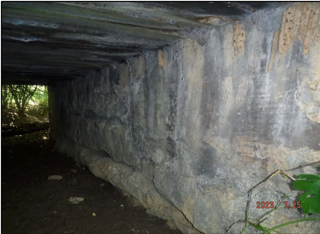
Photo 4: West Abutment (From South)
