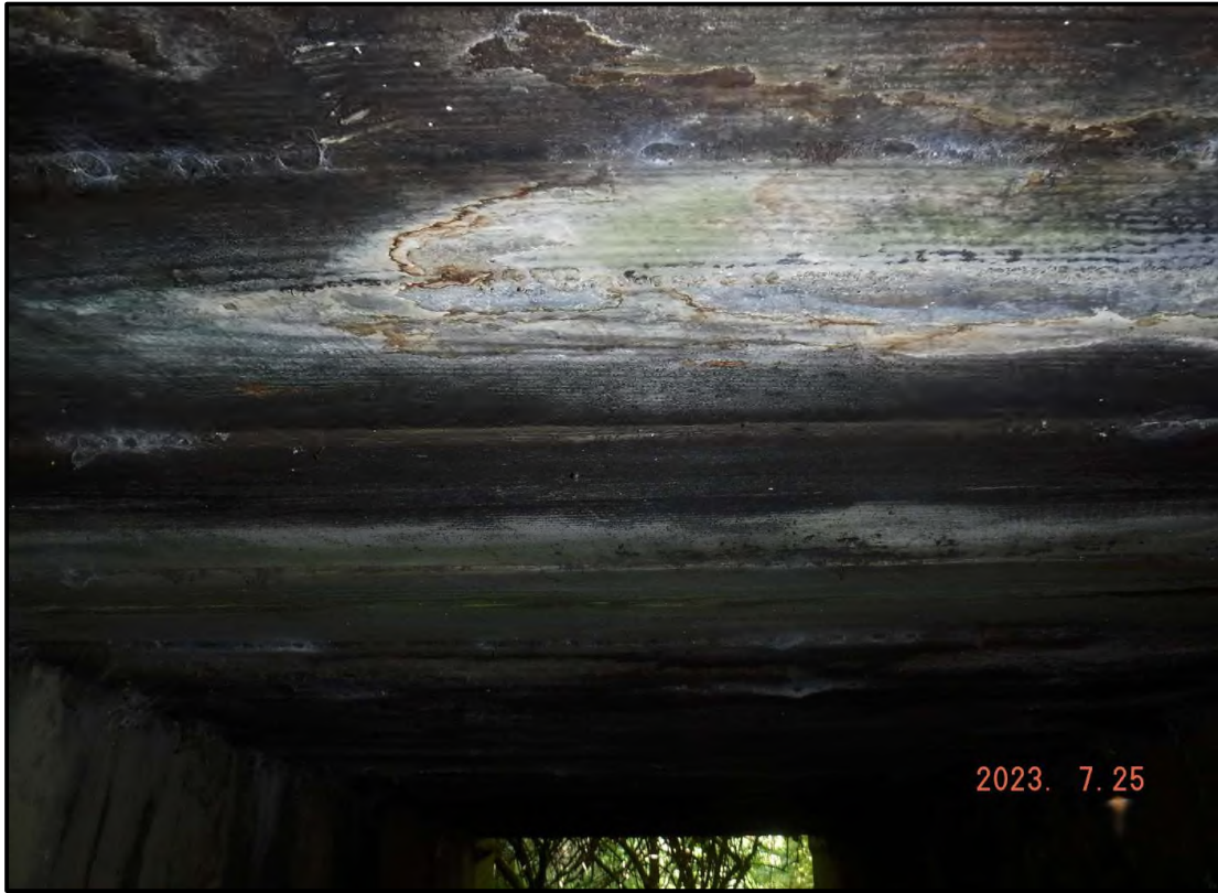
Photo 5: Typical Underside of Timber Slab
