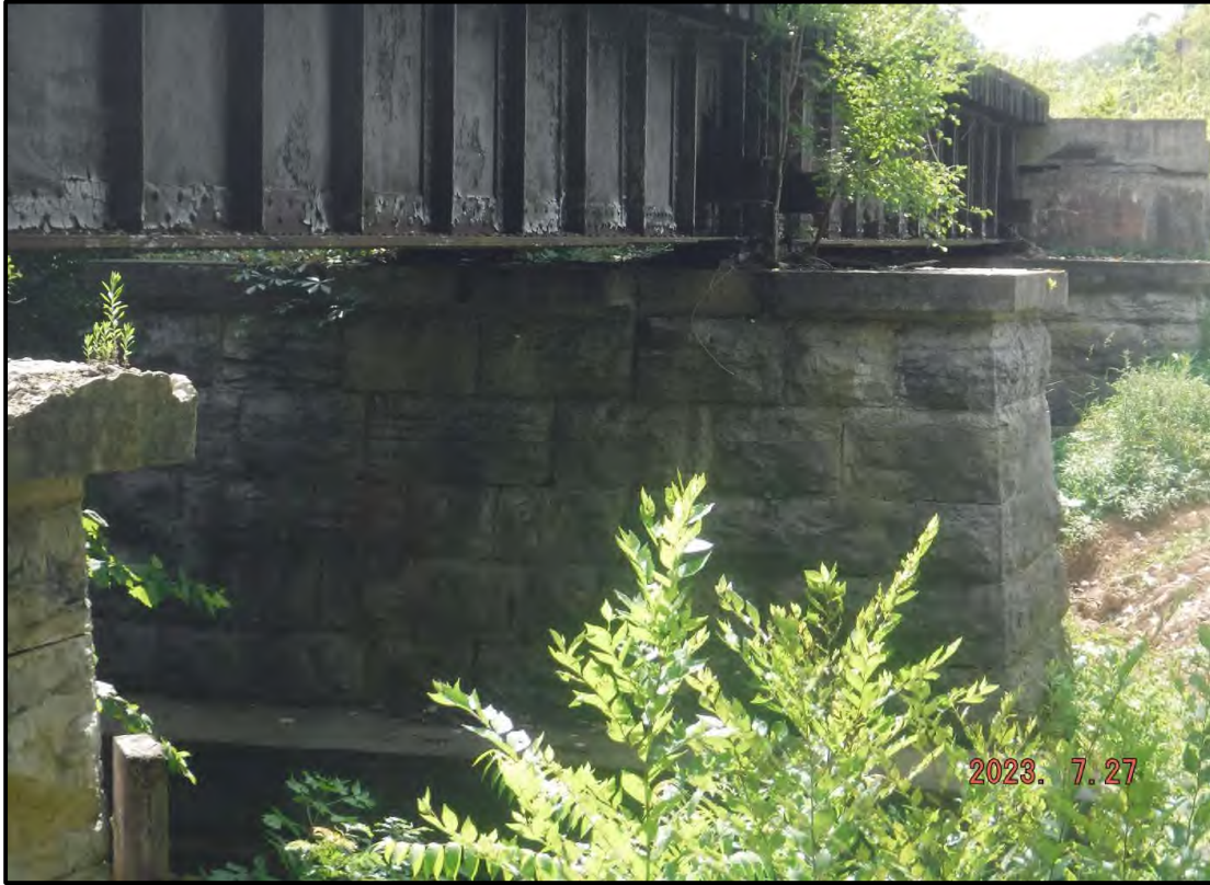
Photo 5: East Side of Pier
