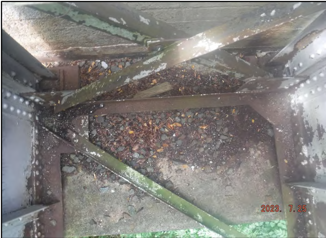
Photo 2: Typical Bridge Seat (West Abutment Shown)
