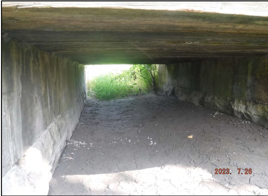
Photo 1: Through Structure (From North)
