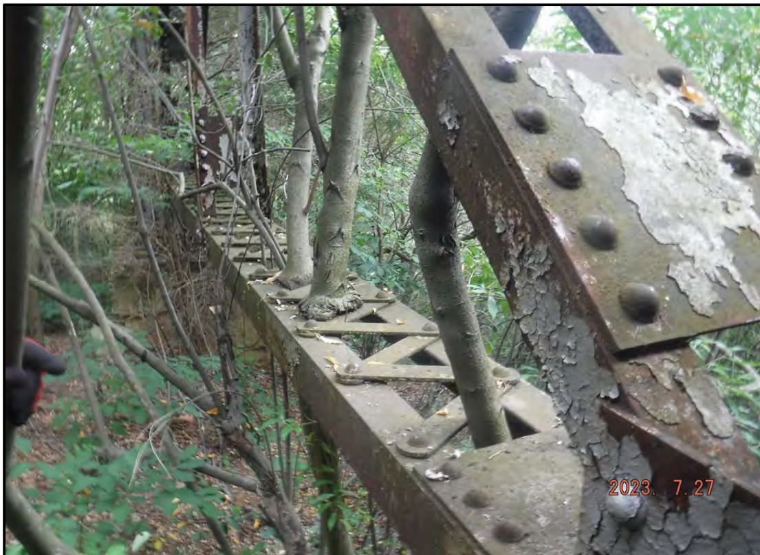
Photo 6: Typical Vegetation in Steel Bent Bracing
