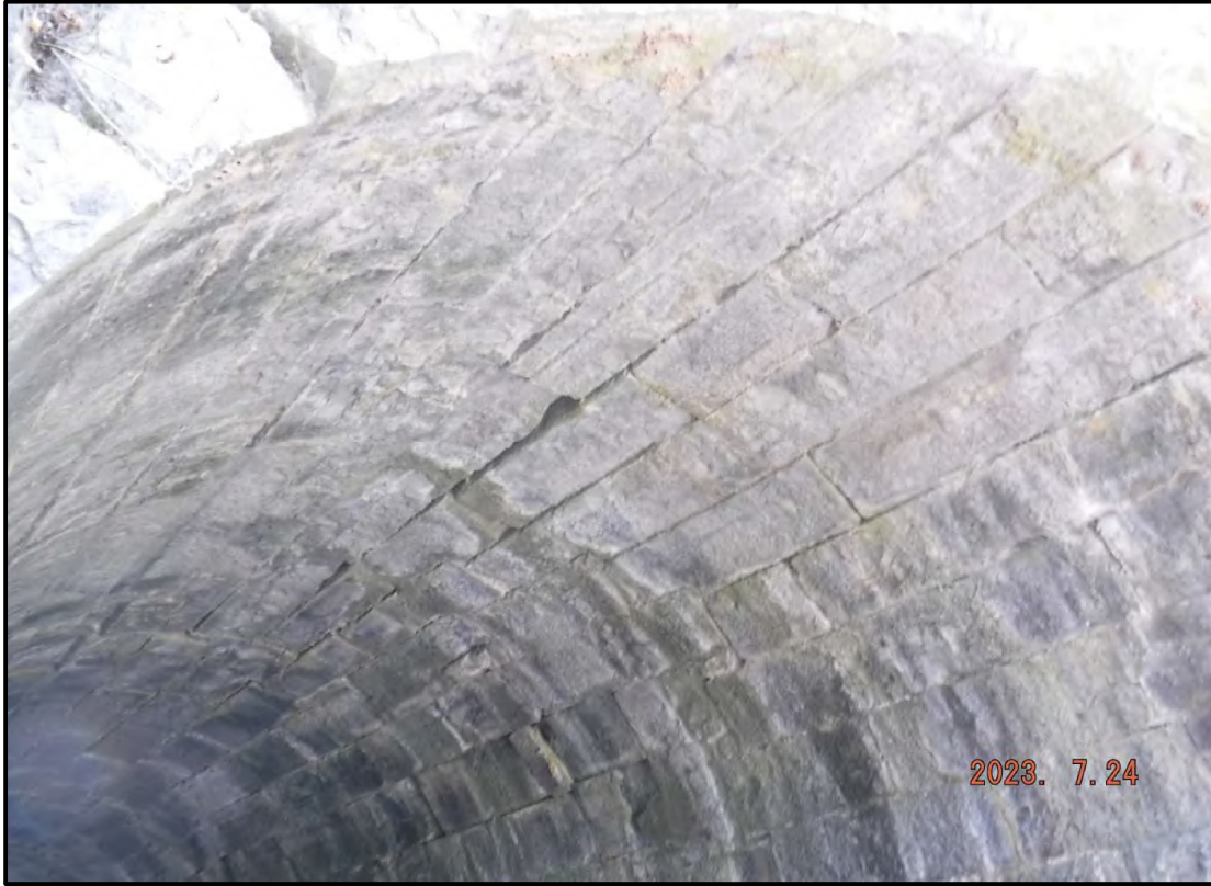
Photo 3: Arch Barrel (From South End)
