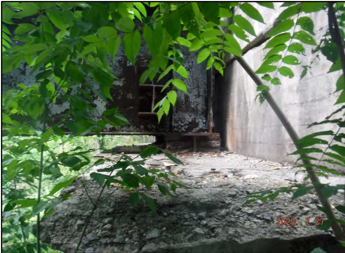
Photo 2: East Abutment Bridge Seat
