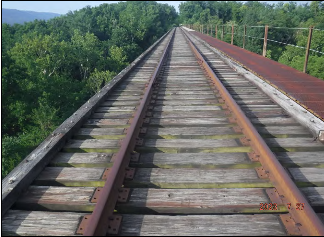
Photo 1: General Condition of Deck (Main Spans)
