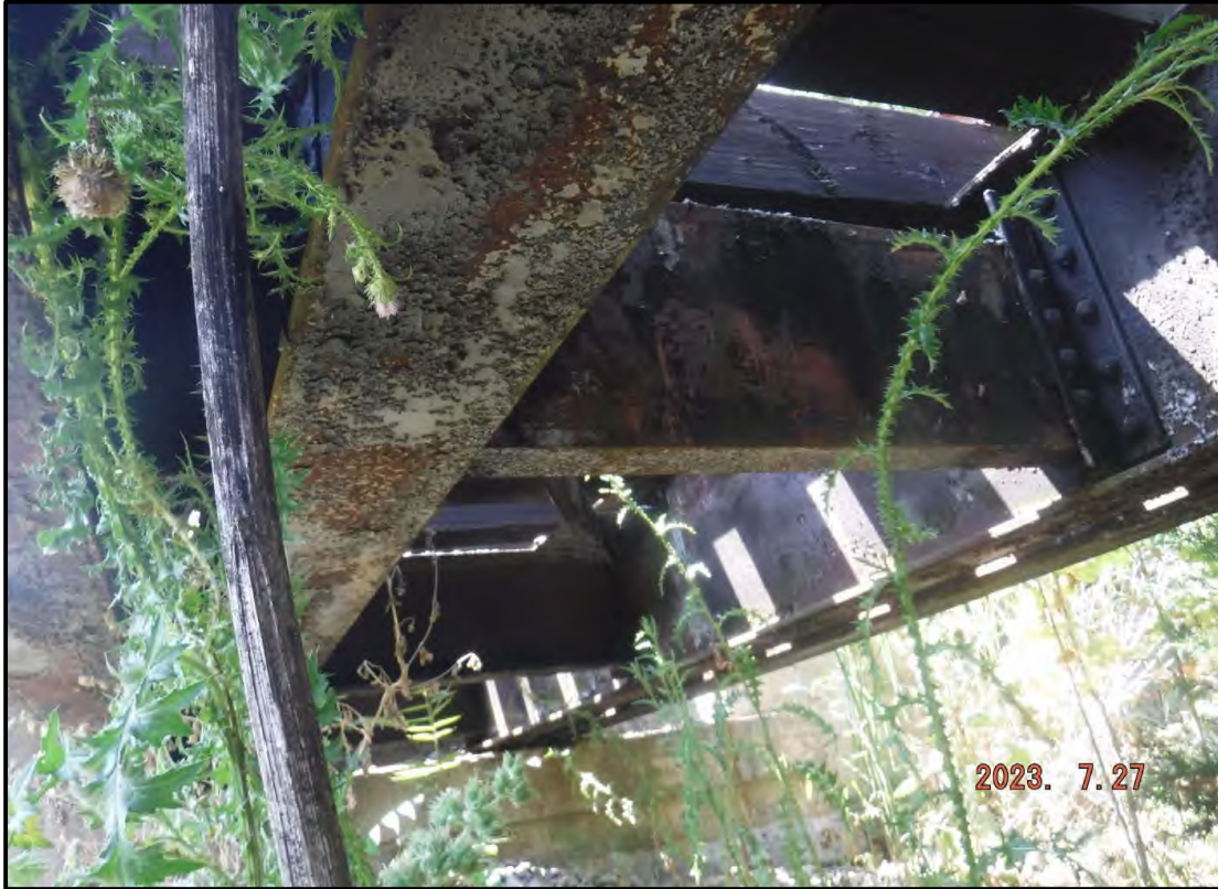
Photo 5: Typical Underside of Span
