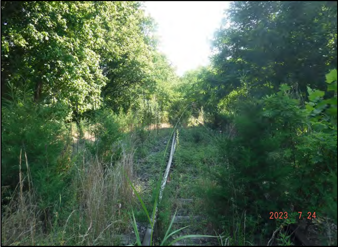
Photo 1: Track on Bridge
