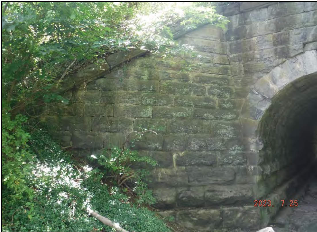
Photo 6: Typical Wingwall (NE Wing Shown)
