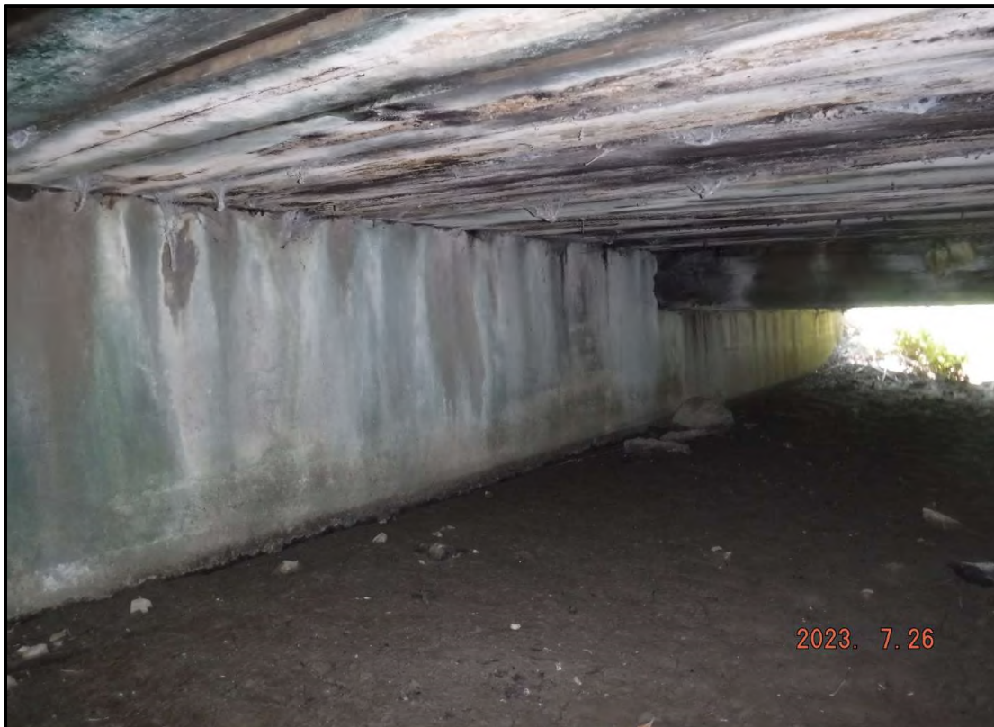
Photo 2: West Abutment (From South)
