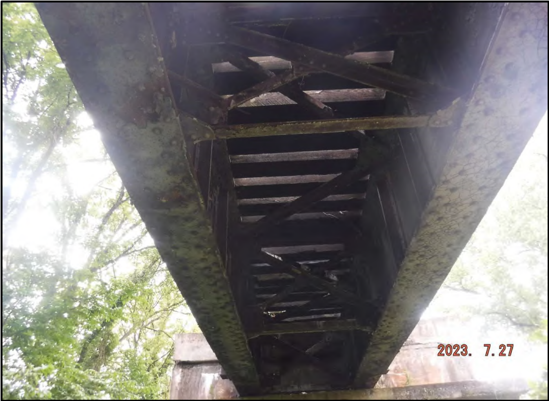
Photo 4: Typical Underside of Span
