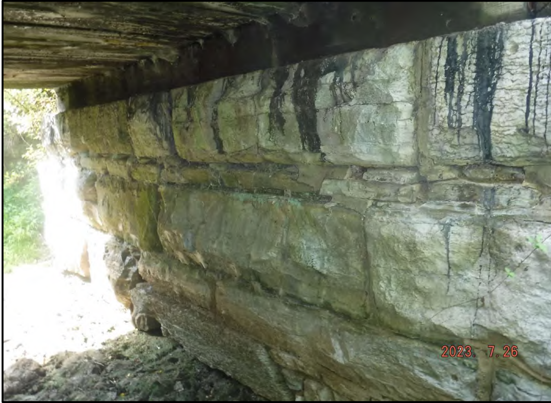
Photo 1: East Abutment (From South)
