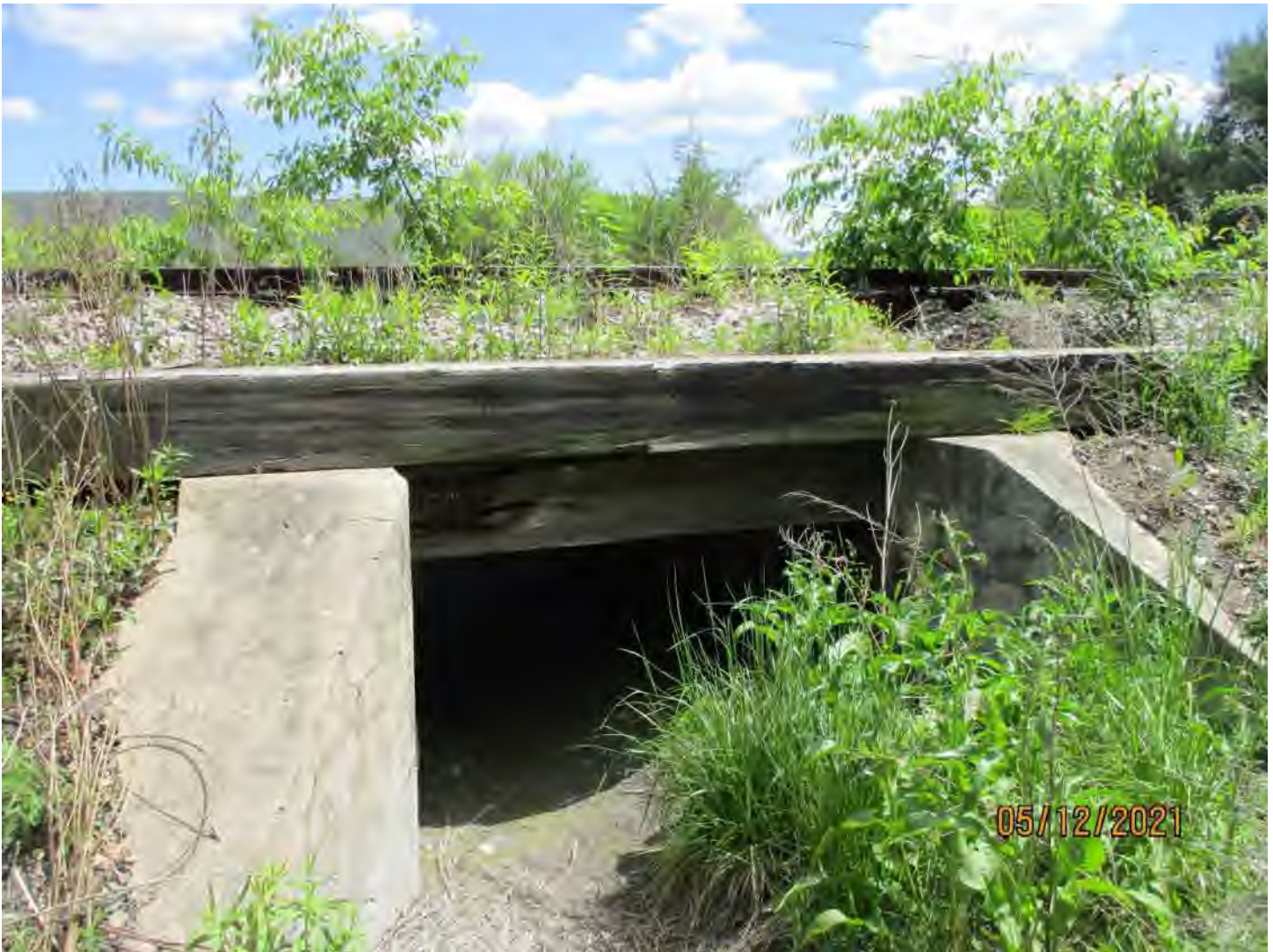
Asset 8452 over Unnamed Drainage Crossing N 38° 45' 48.99", W 78° 37' 33.91" Single Barrel Culvert, 17'-0"
