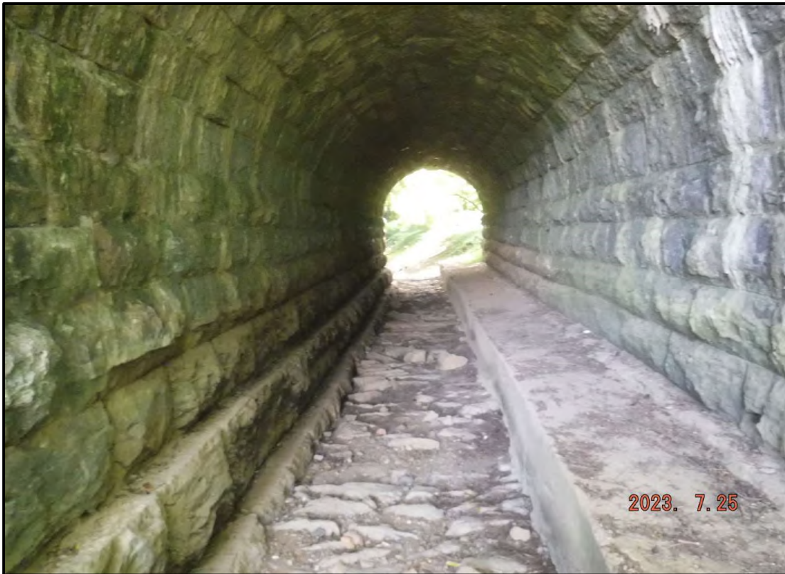
Photo 4: Through Stone Arch (From North)
