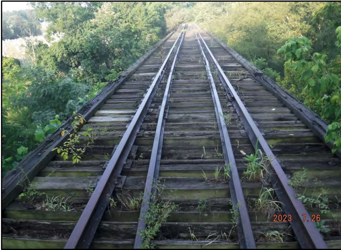
Photo 1: General Condition of Timber Tie Deck
