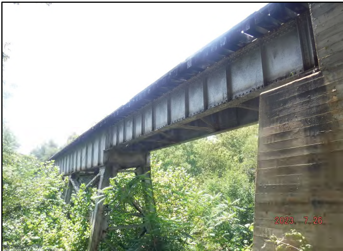
Photo 2: Typical Girders (South Side from East)
