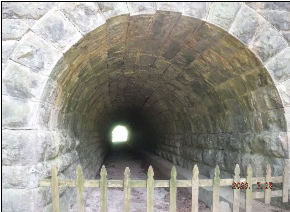
Photo 2: Through Stone Arch (From North)
