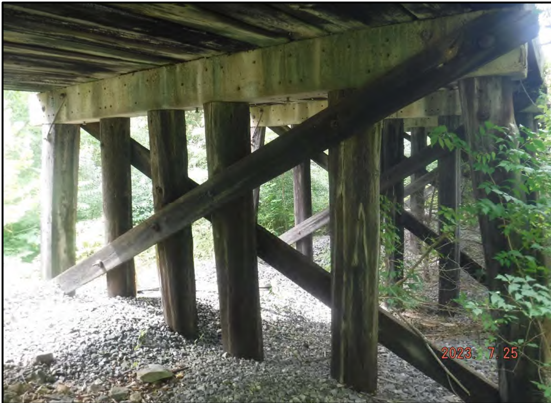
Photo 4: Typical Timber Pile Bent
