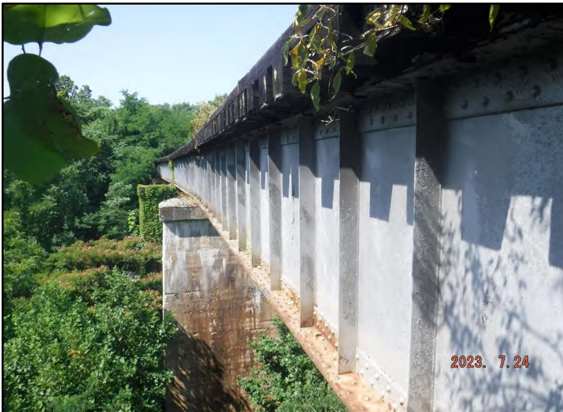
Photo 6: Typical Condition of Girders (From SE looking West)
