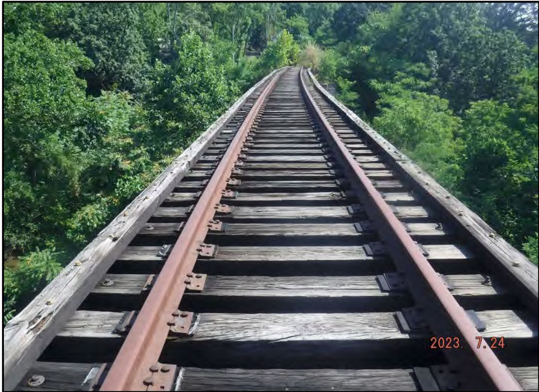
Photo 1: General Condition of Timber Tie Deck
