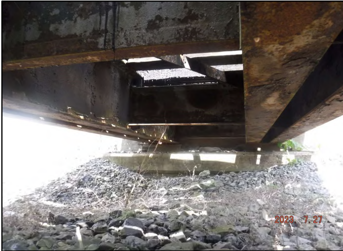
Photo 5: Typical Underside of Span
