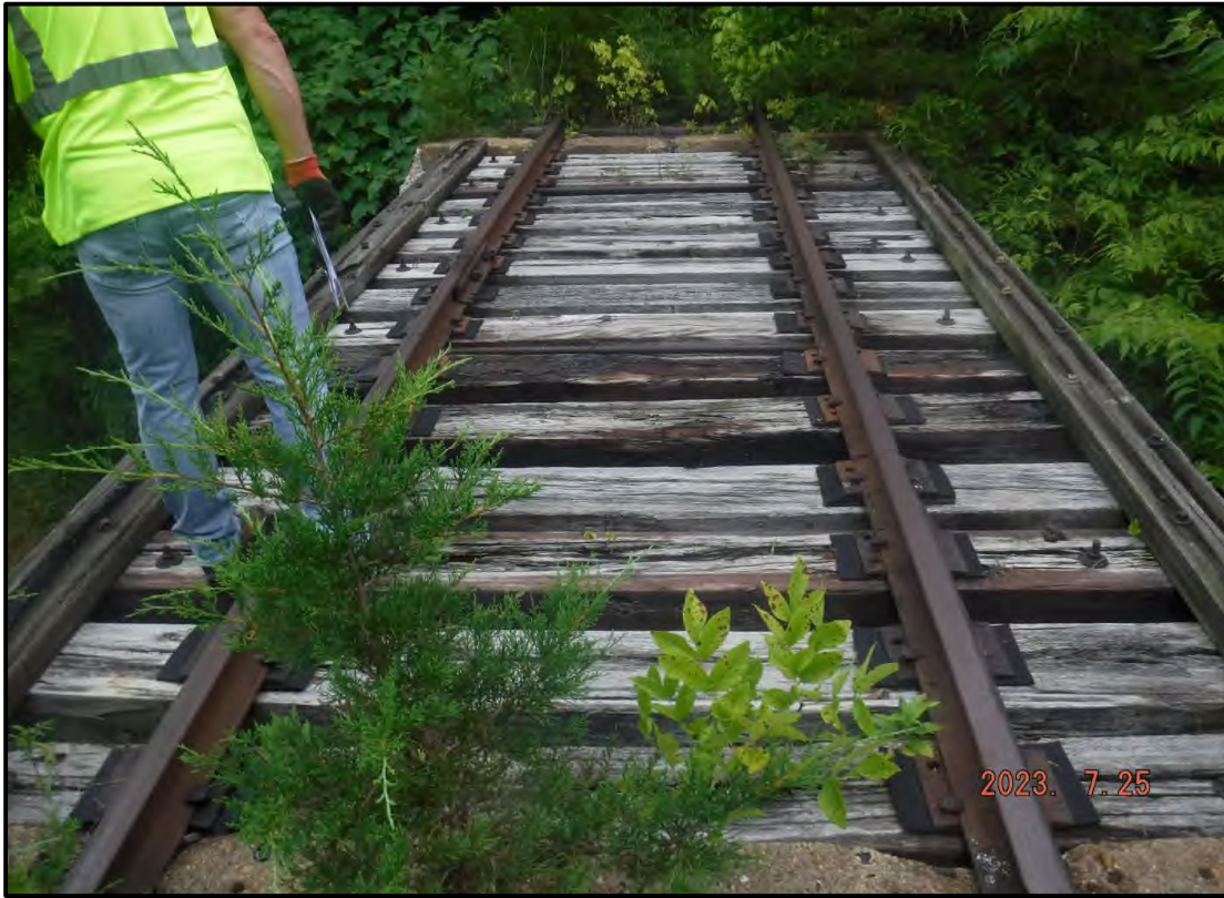
Photo 1: General Condition of Bridge Deck
