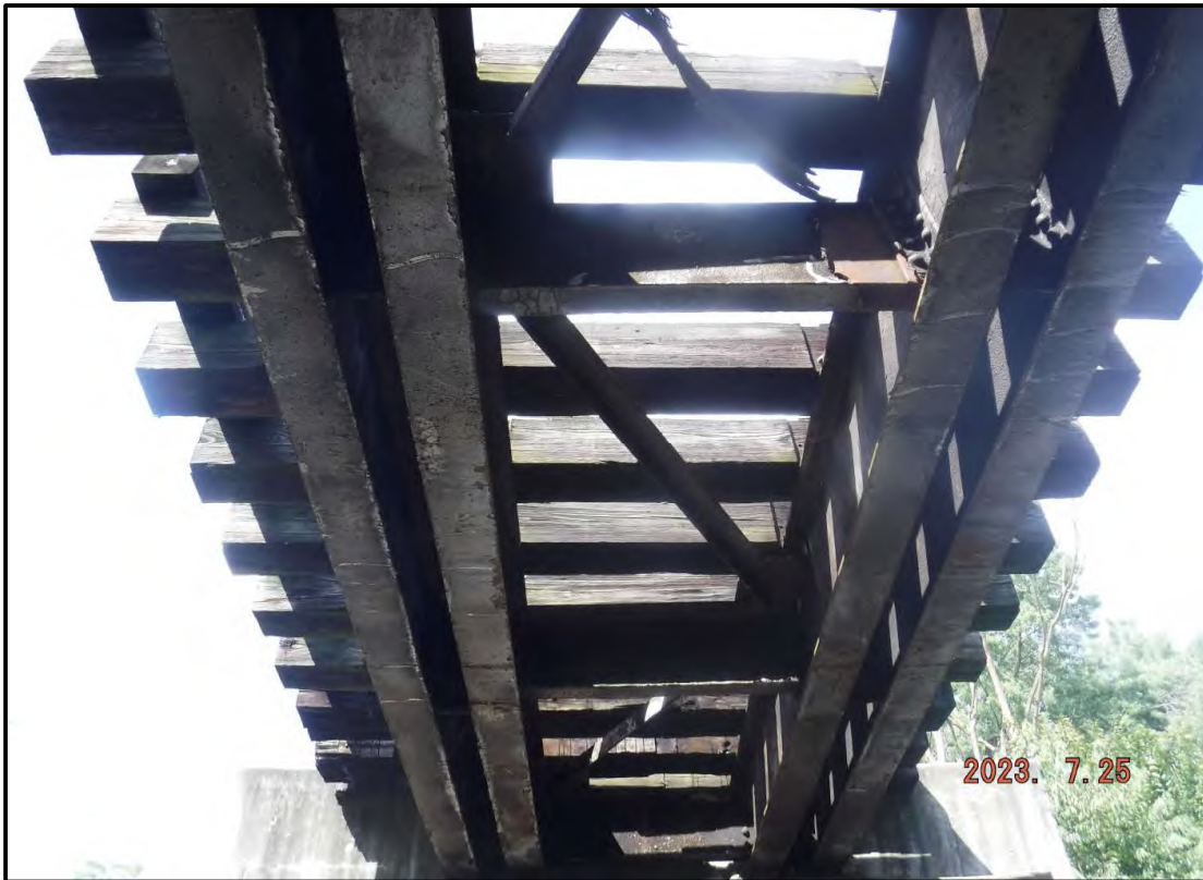
Photo 6: Underside of Span
