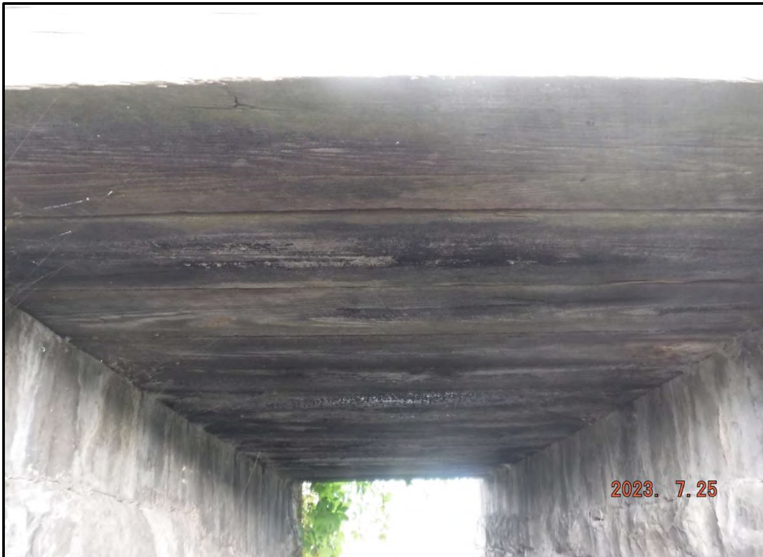
Photo 4: Underside of Timber Slab
