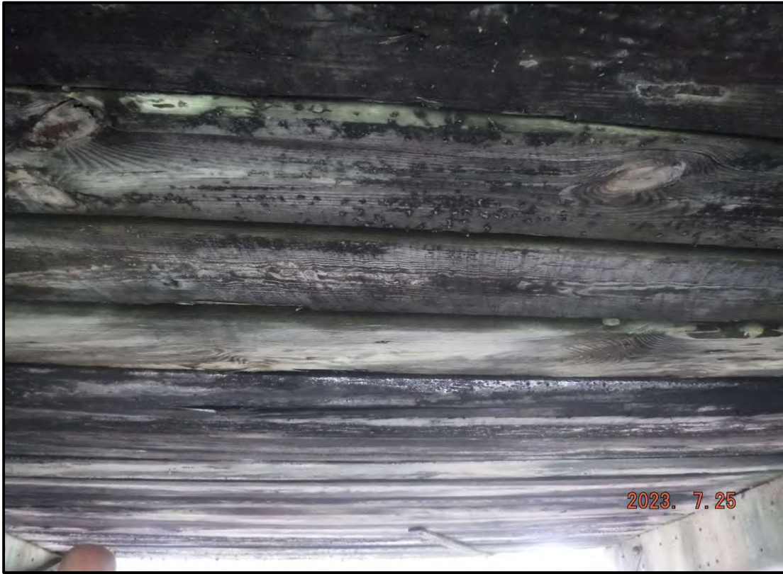
Photo 5: Typical Underside of Timber Slab
