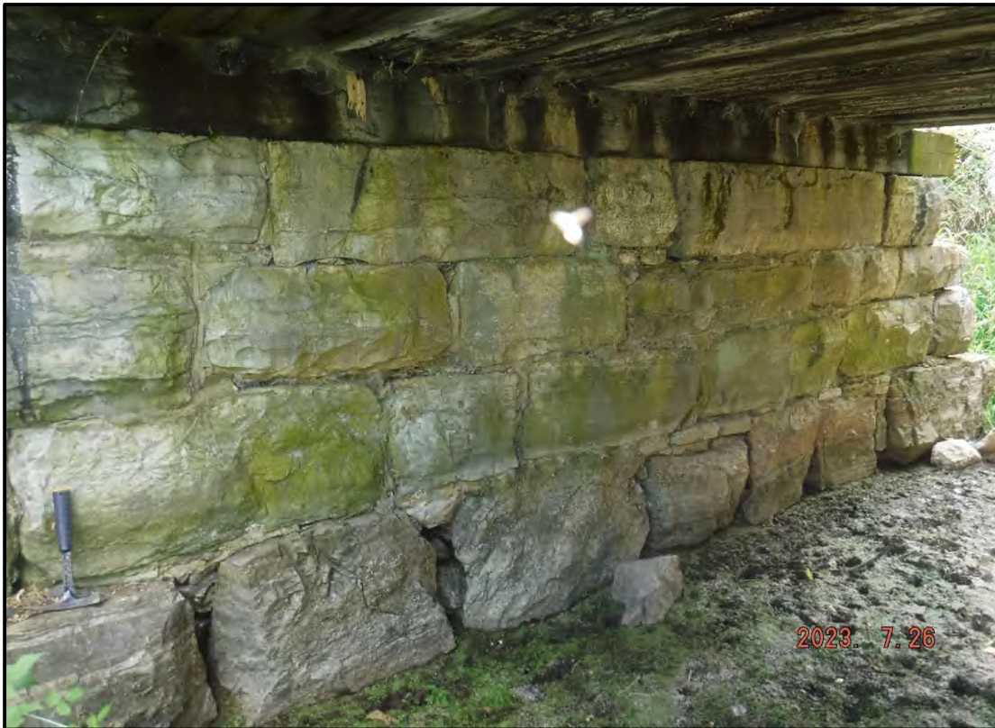
Photo 2: West Abutment (From South)
