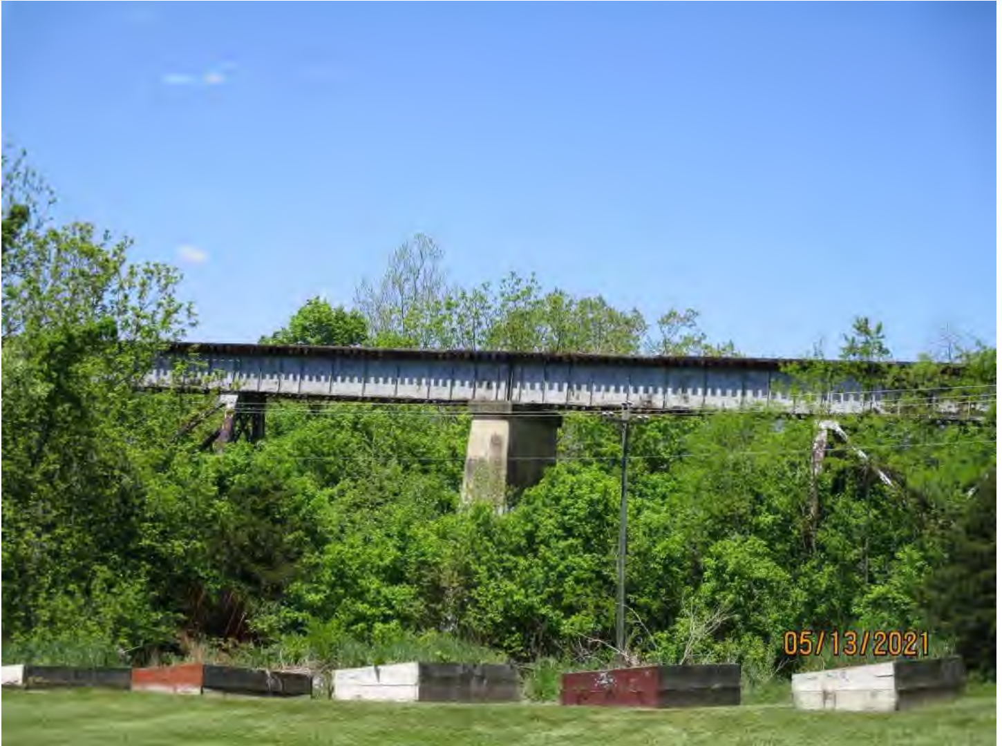
Asset 6765 over Toms Brook N 38° 56' 46.70", W 78° 26' 33.18" Twelve Span Steel Girder Bridge, 510'-0"
