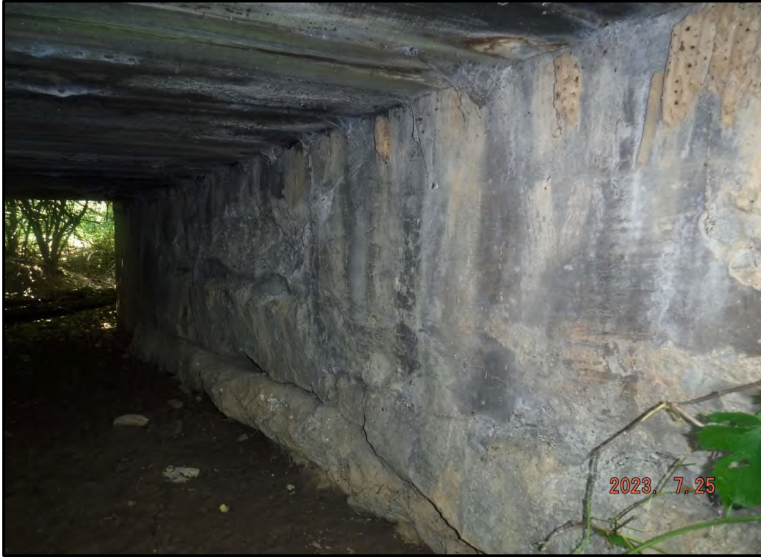
Photo 3: East Abutment (From South)
