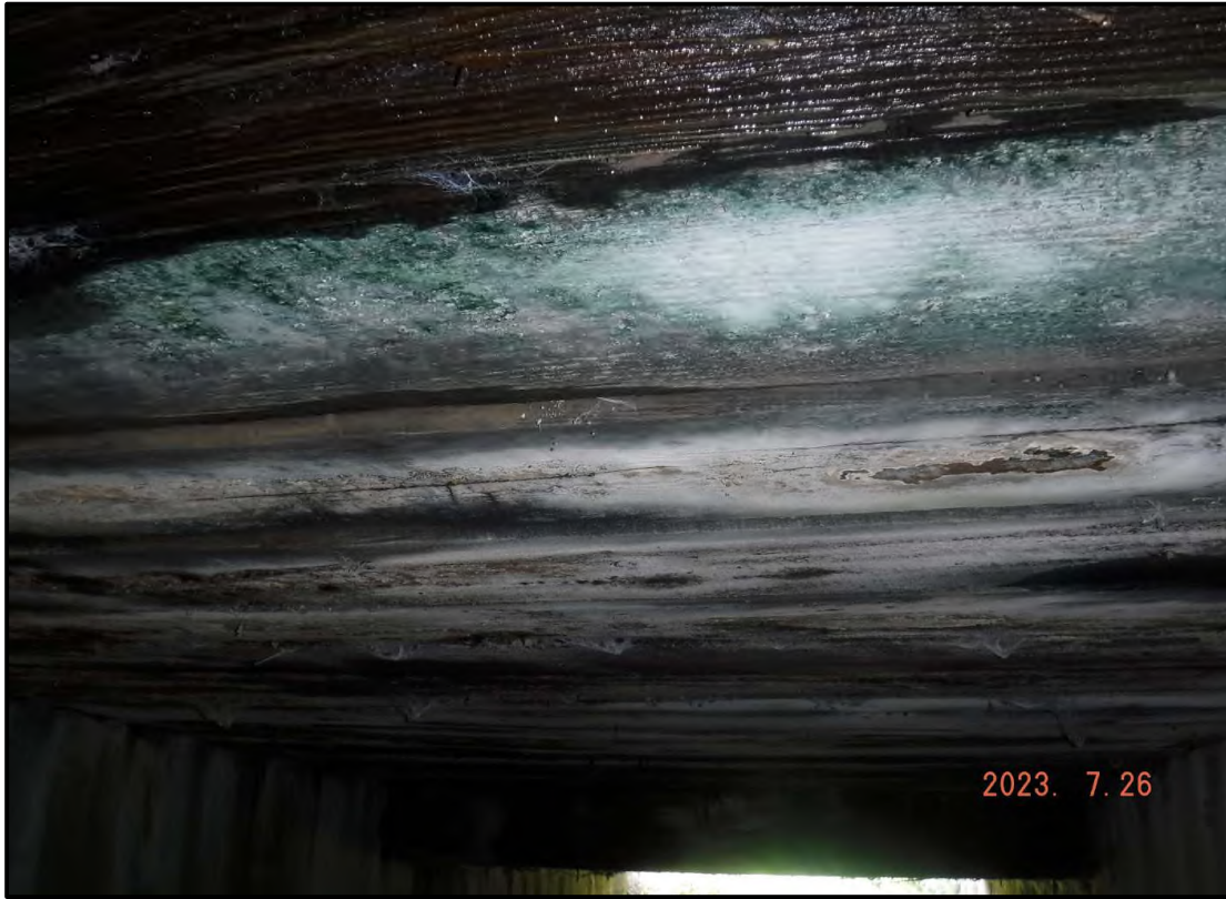
Photo 3: Typical Timber Slab (From South)
