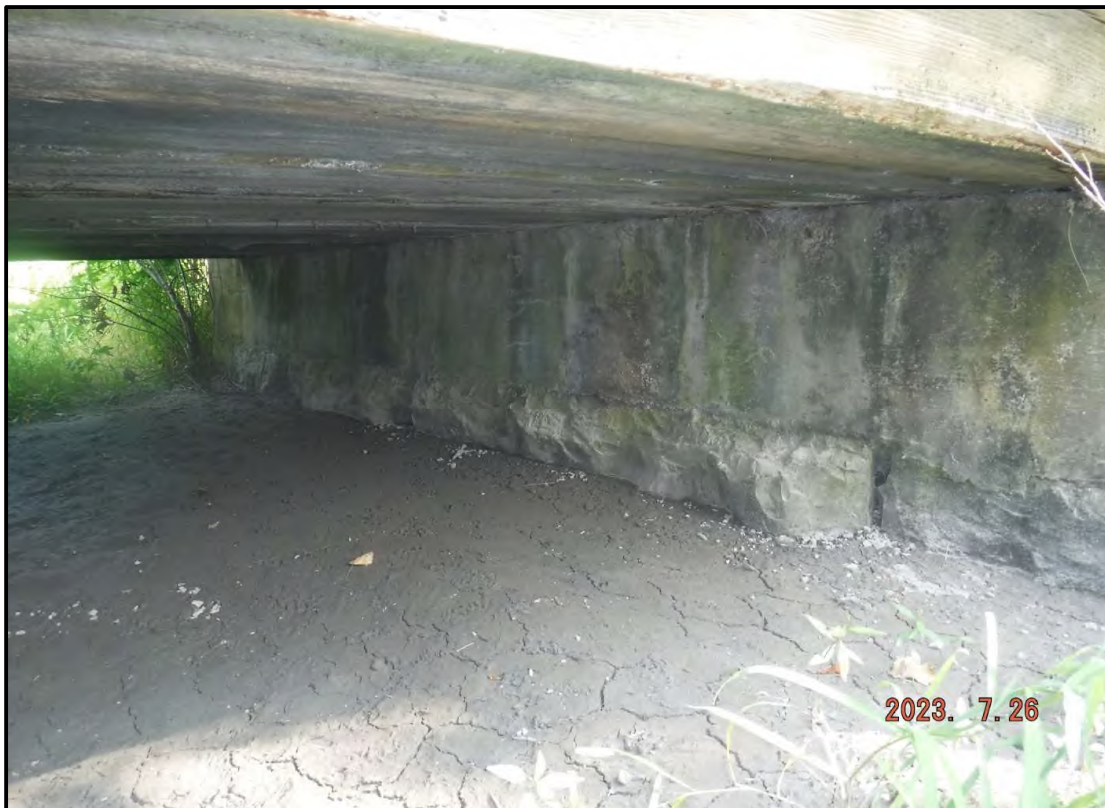
Photo 2: West Abutment (From North)
