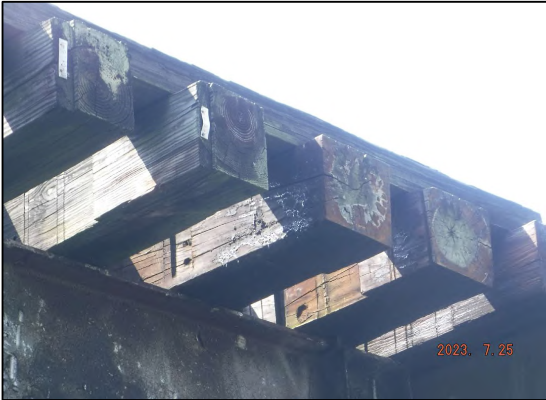
Photo 3: General Condition of Timber Tie Deck
