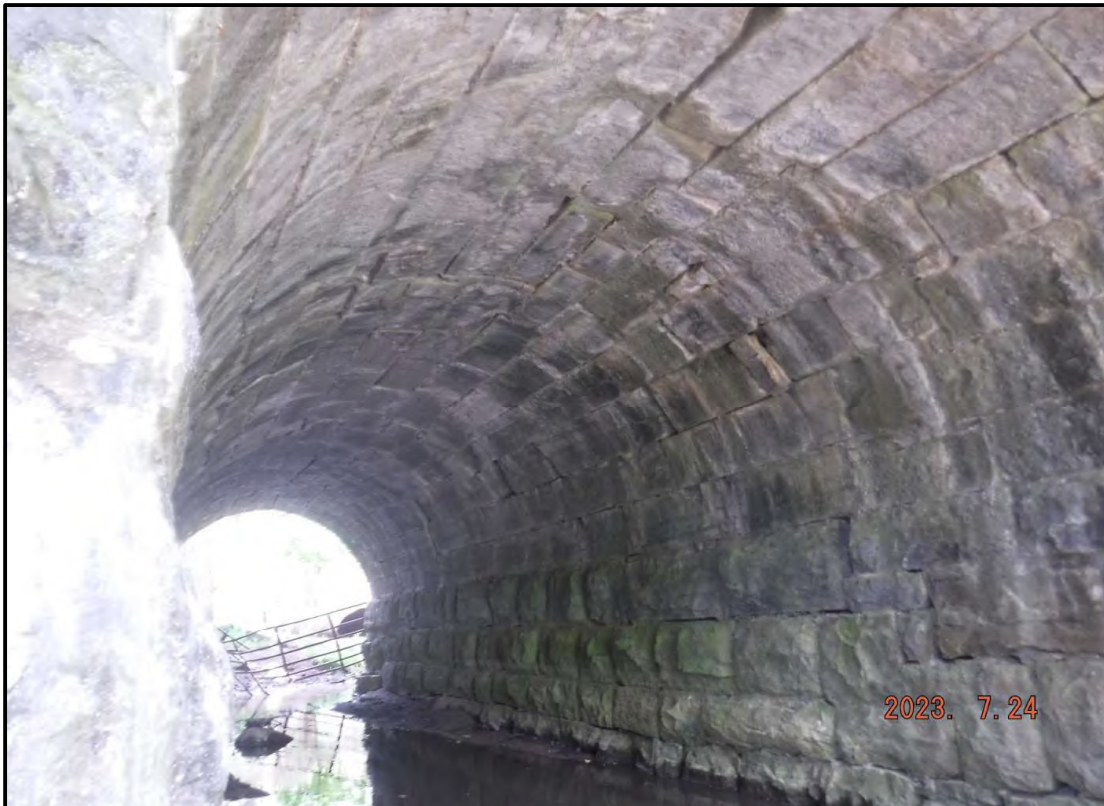
Photo 2: Through Arch (From South End)
