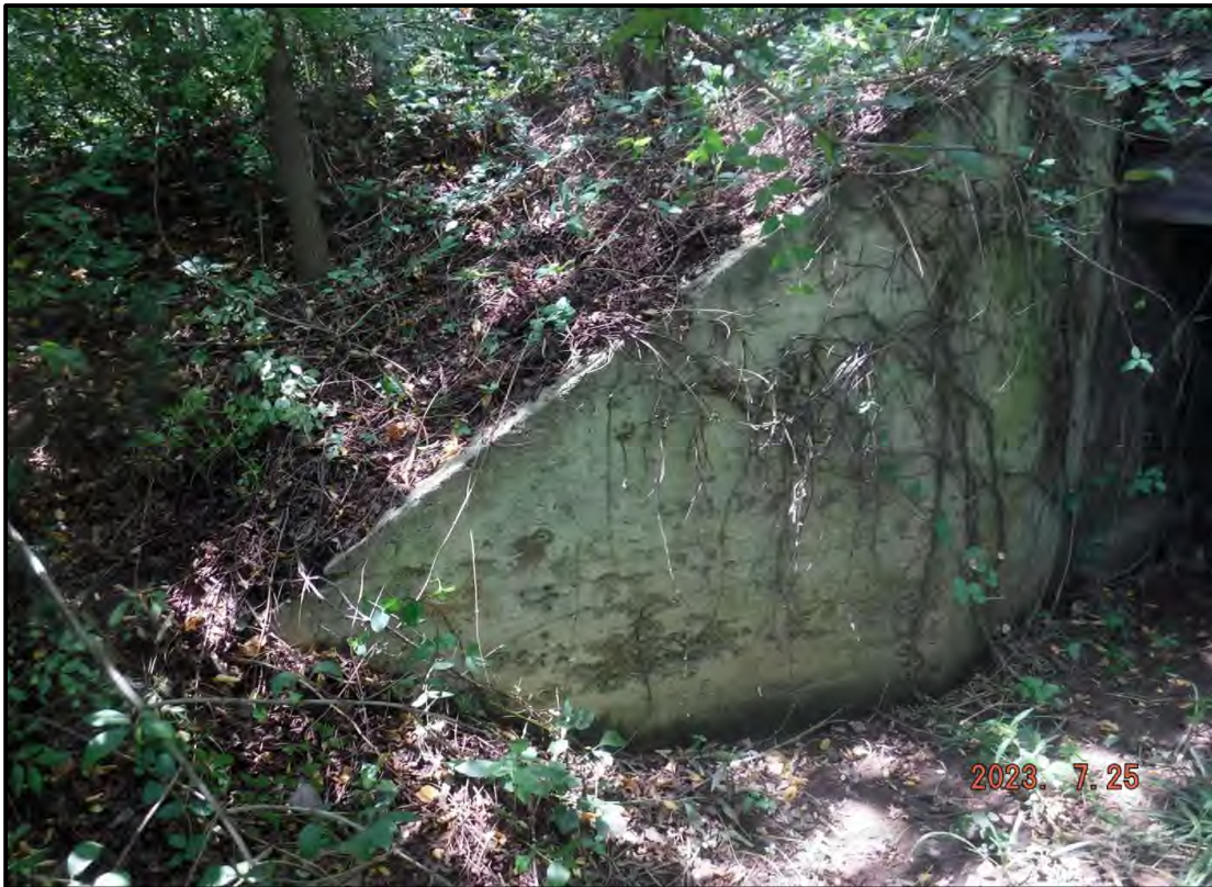
Photo 2: Typical Wingwall (SW Wing Shown)
