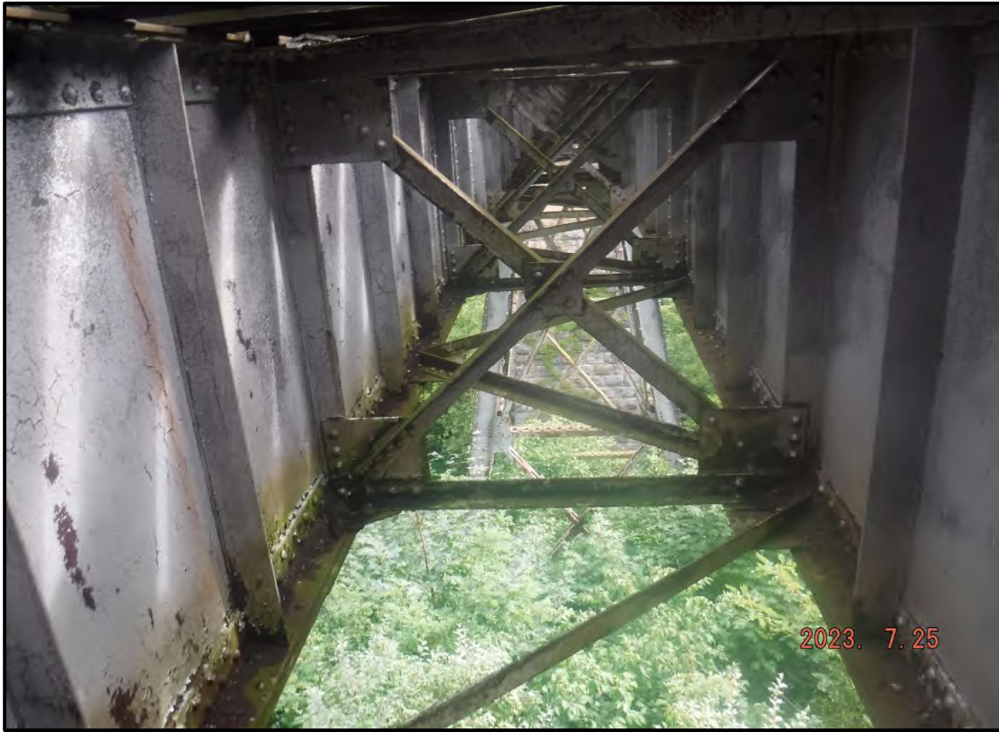
Photo 3: Through Girders (From West Abutment)
