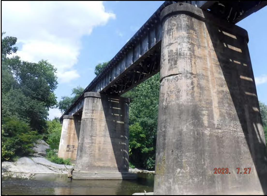
Photo 5: Piers (From NW)
