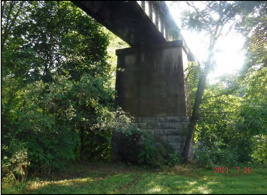
Photo 5: Typical Pier (West Side of Pier 2 Shown)
