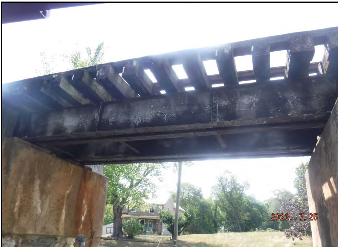
Photo 2: South Elevation of Girders
