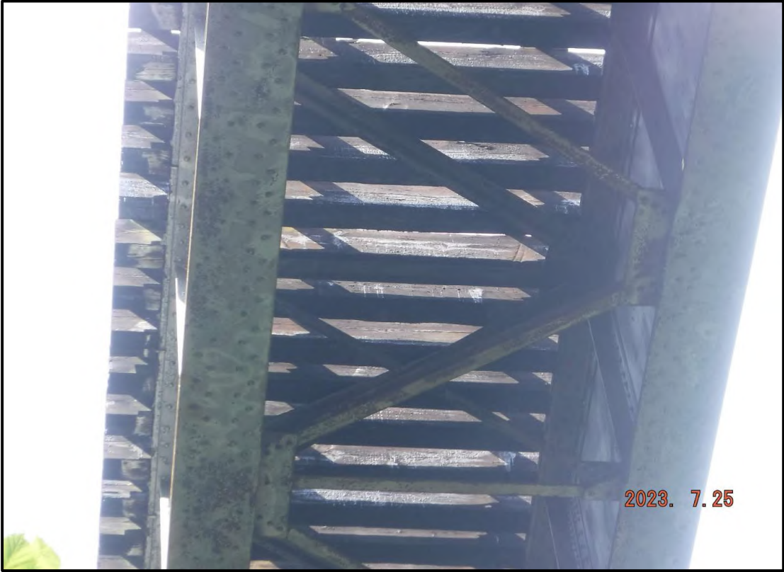
Photo 1: General Condition of Timber Tie Deck
