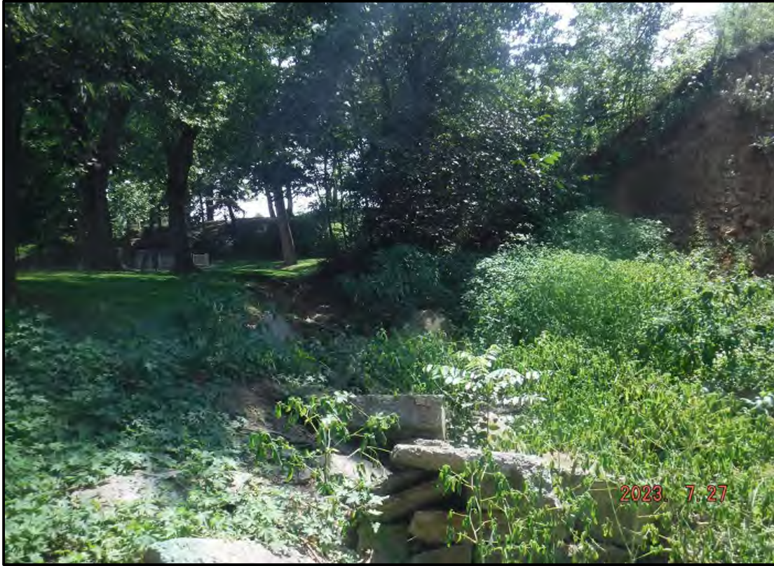
Photo 3: Looking West Up Drainage Ditch at SW Corner of Structure
