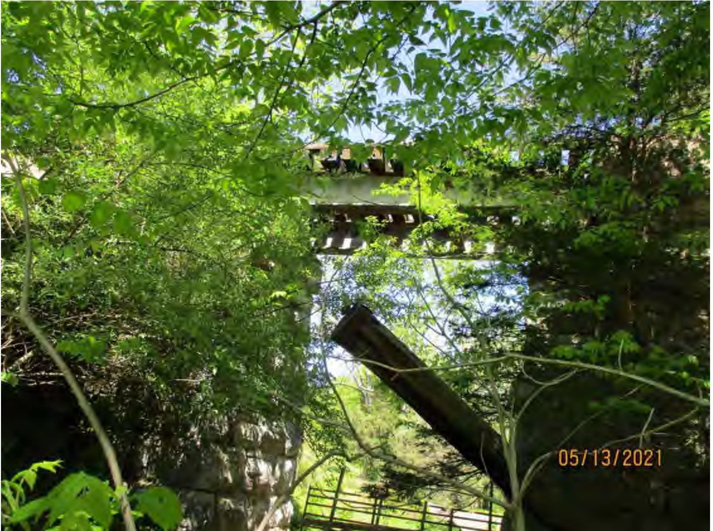
Asset 6824 over Jordan Run N 38° 56' 28.06", W 78° 27' 4.34" Single Span Steel Girder Bridge, 19'-1"
