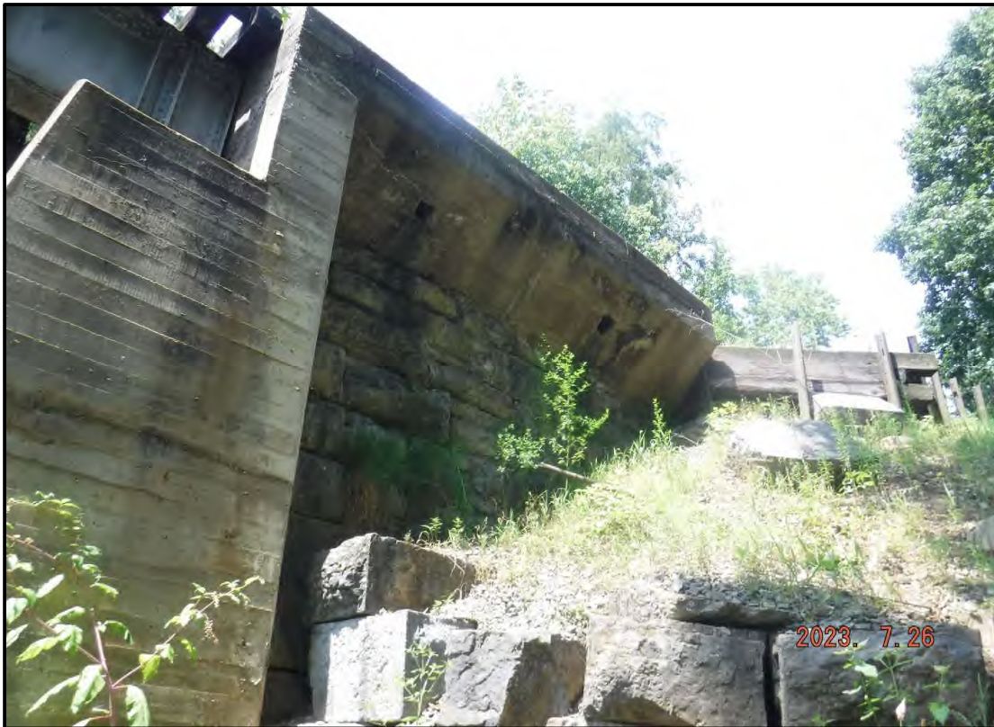
Photo 6: East Approach Trough Structure Behind East Abutment
