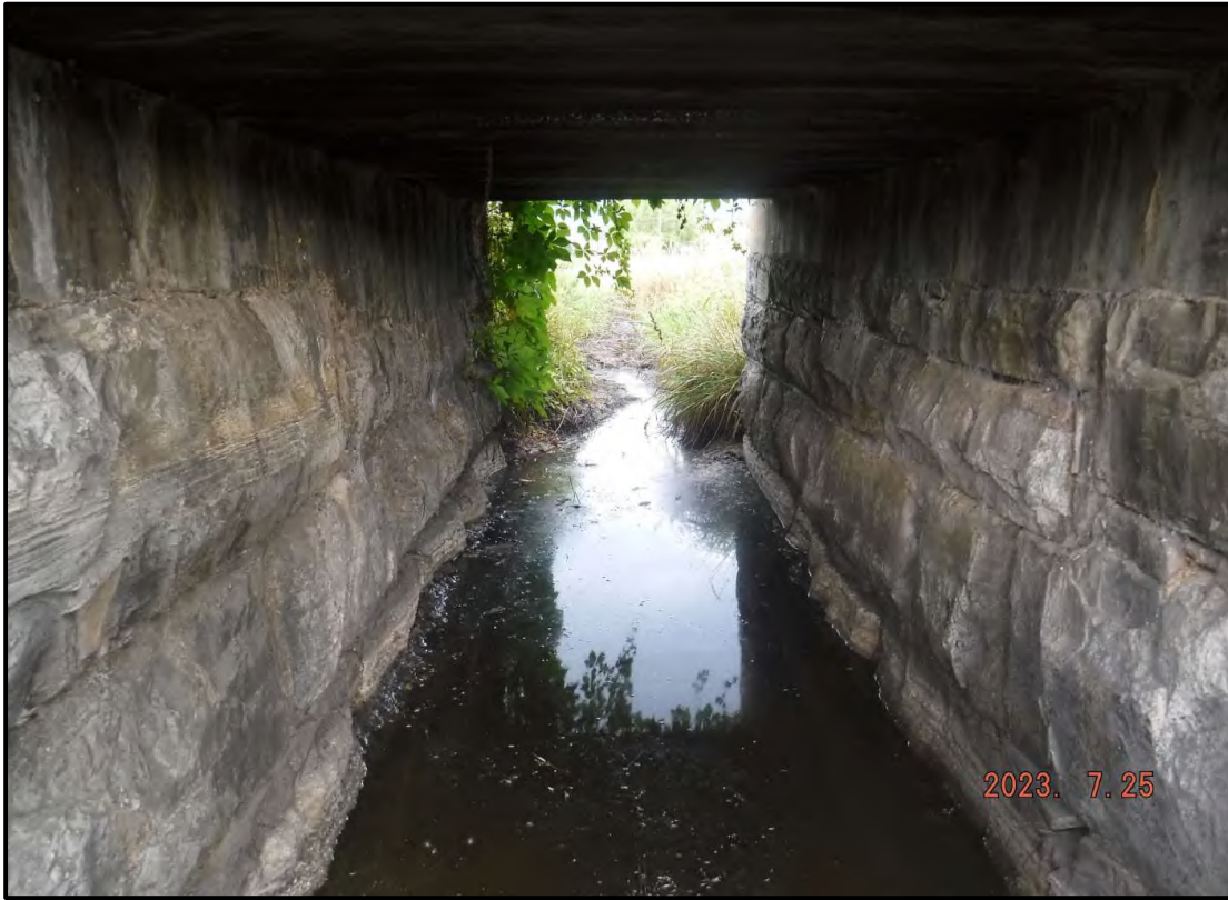
Photo 3: Through Structure (From North)
