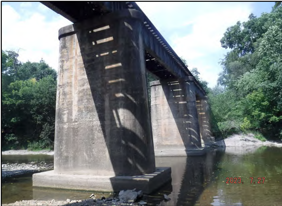
Photo 4: Piers (From SW)
