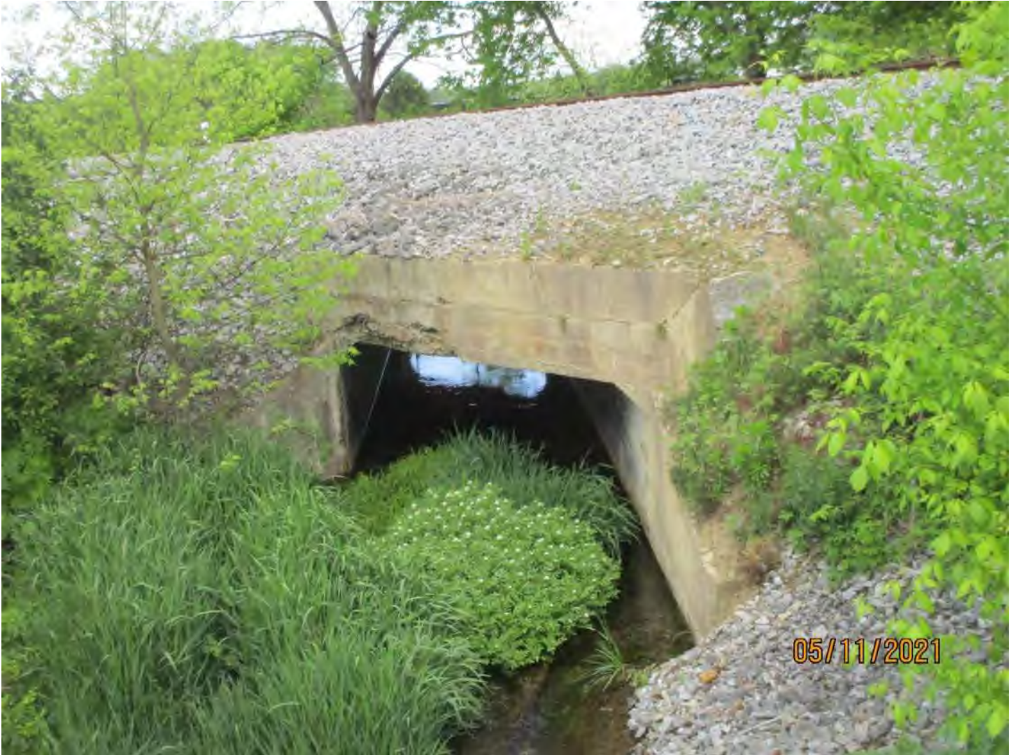
Asset 9540 over Unnamed Drainage Crossing N 38° 38' 48.52", W 78° 44' 34.44" Single Barrel Concrete Culvert, 41'-0"
