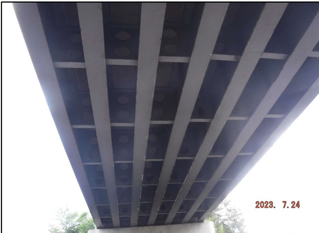
Photo 4: Underside of Typical Span (Span 2 Shown)
