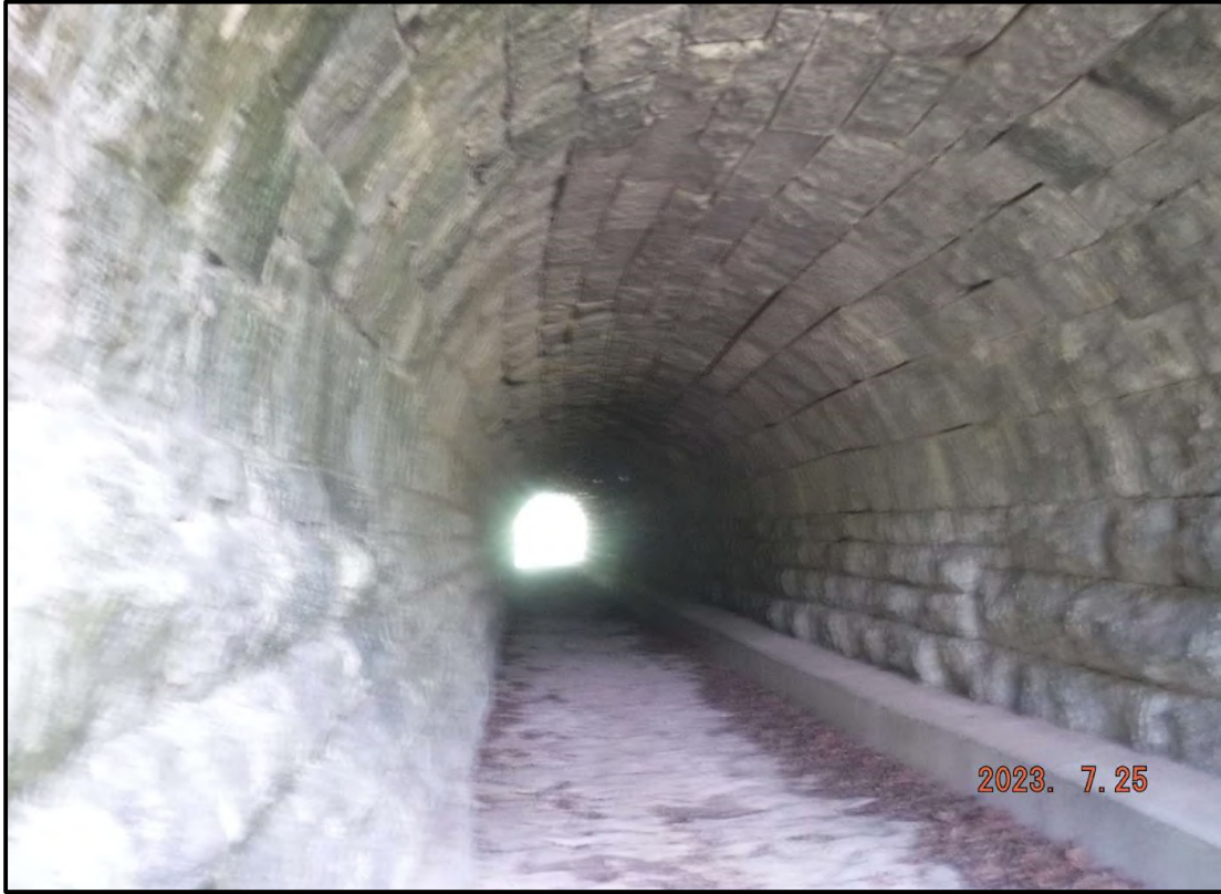
Photo 3: Through Stone Arch (From South)
