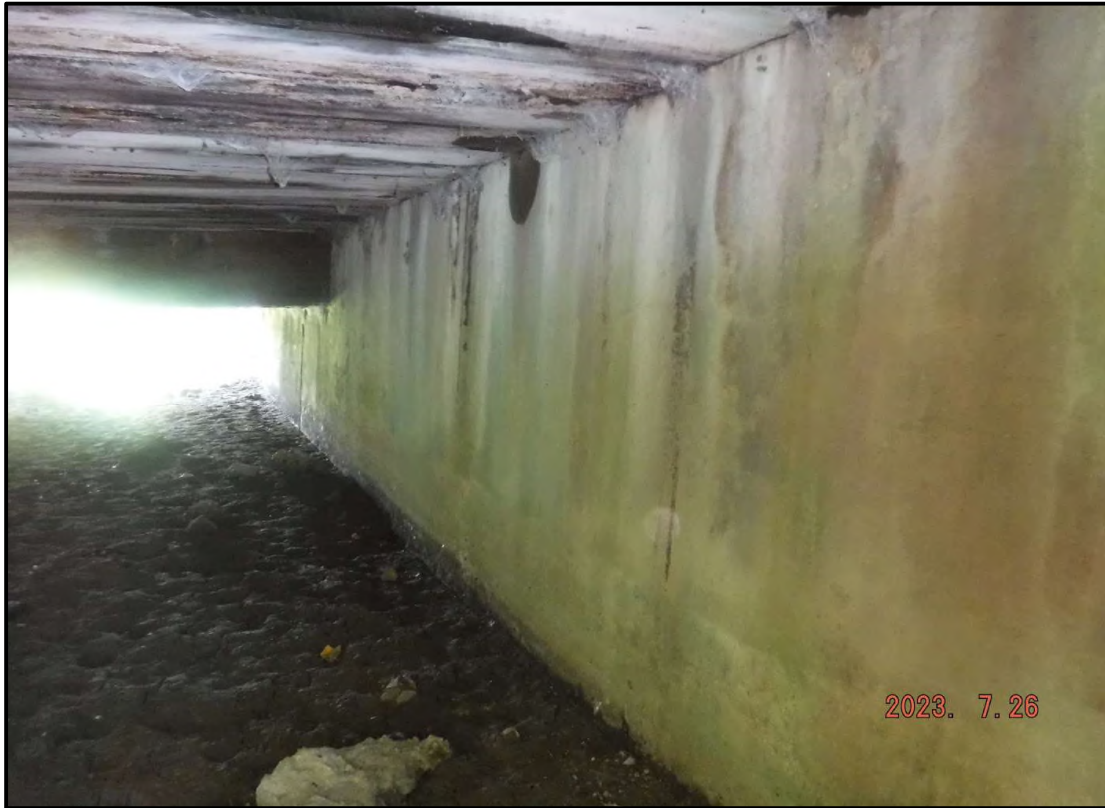
Photo 1: East Abutment (From South)
