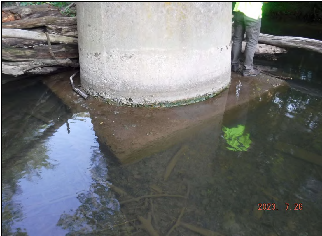
Photo 6: Typical Exposed Footing (Steel Bent Tower)
