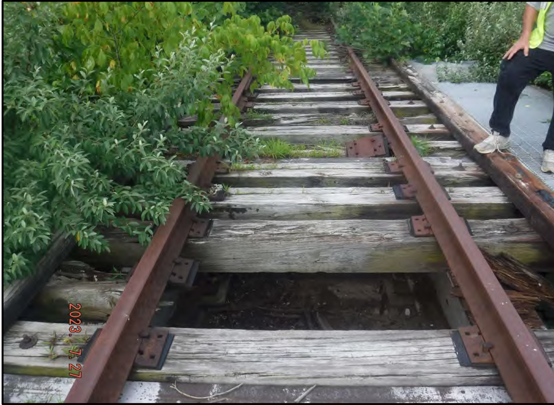
Photo 3: General Condition of Deck (Approach Spans, West Shown)
