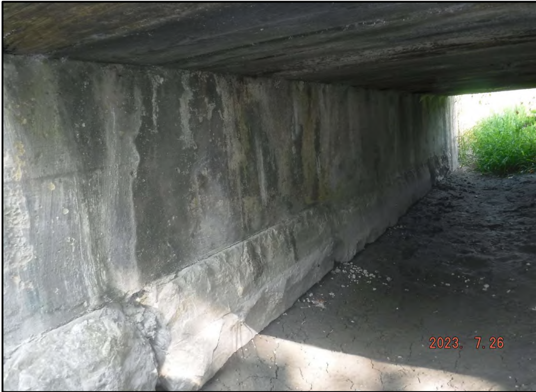
Photo 3: East Abutment (From North)
