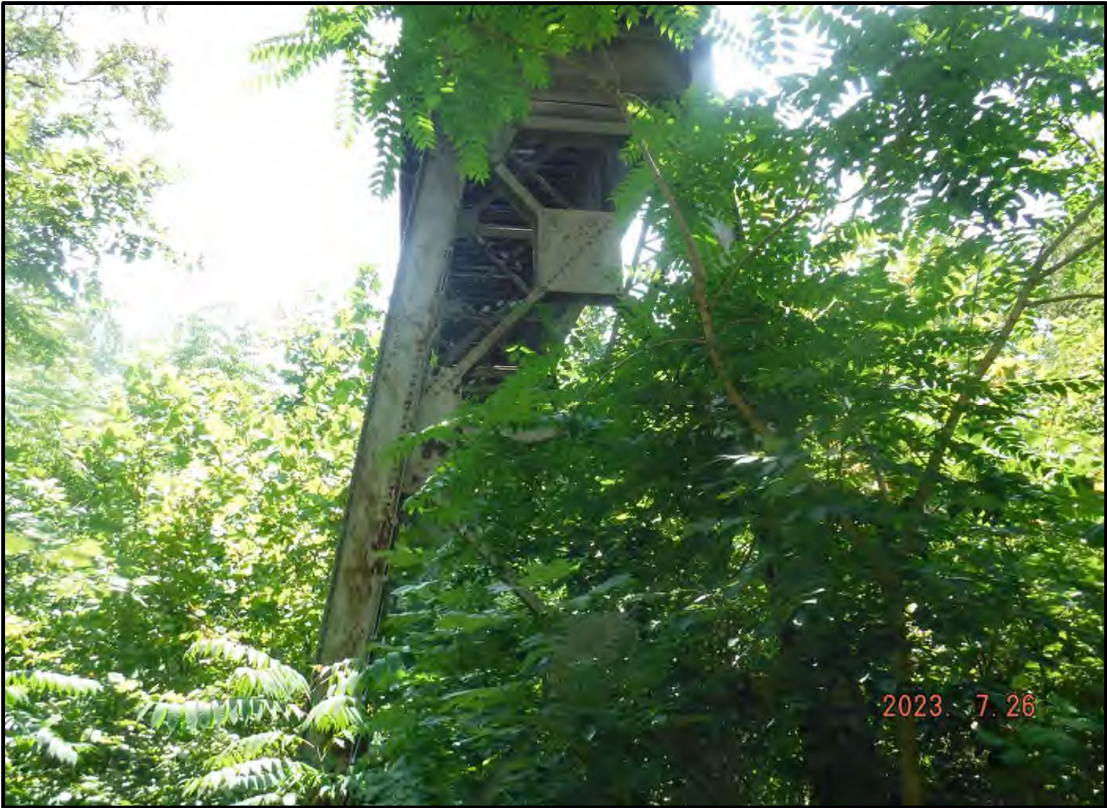
Photo 4: Typical Steel Bent Tower
