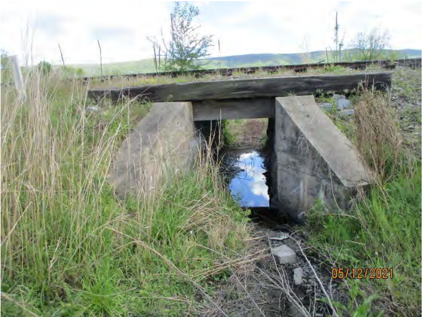
Asset 8438 over Unnamed Drainage Crossing N 38° 45' 54.63", W 78° 37' 28.07" Single Barrel Culvert, 16'-6"
