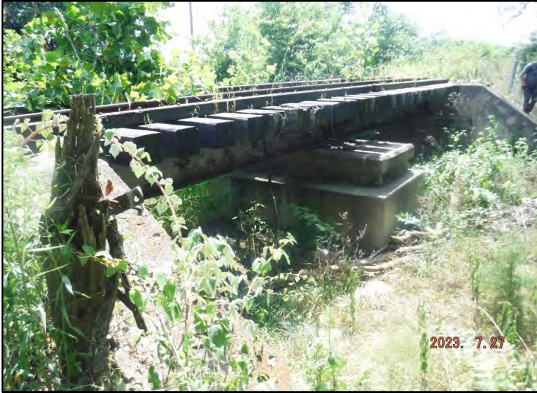
Photo 1: General Condition of Timber Tie Deck
