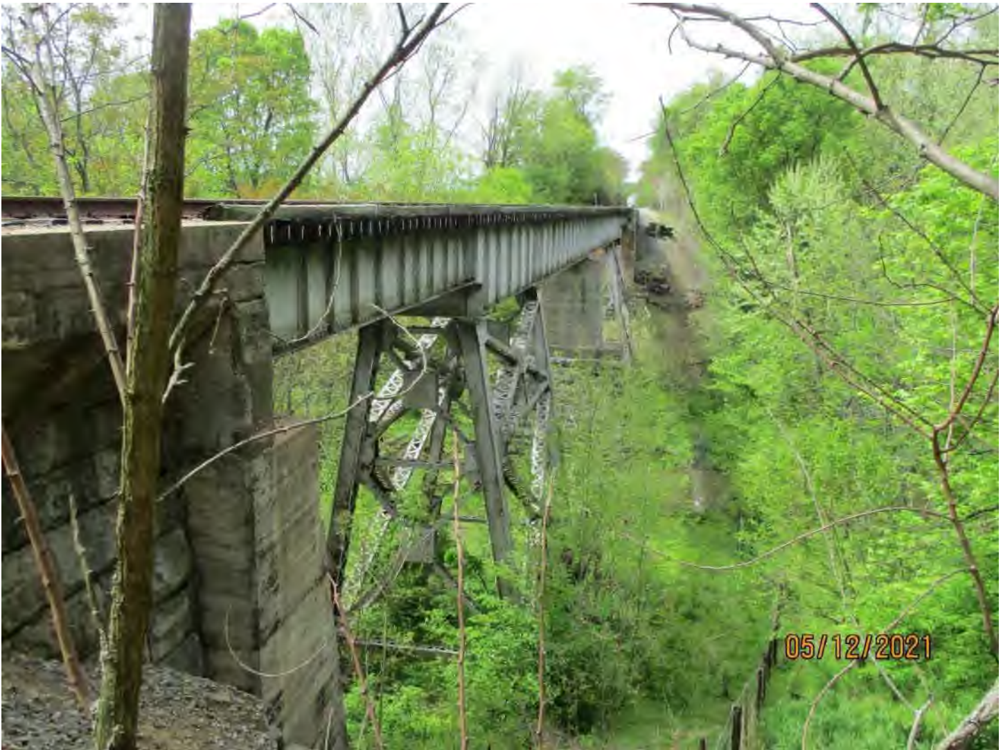
Asset 8984 over Holmans Creek N 38° 41' 53.68", W 78° 40' 32.78" Six Span Steel Girder Bridge, 310'-0"
