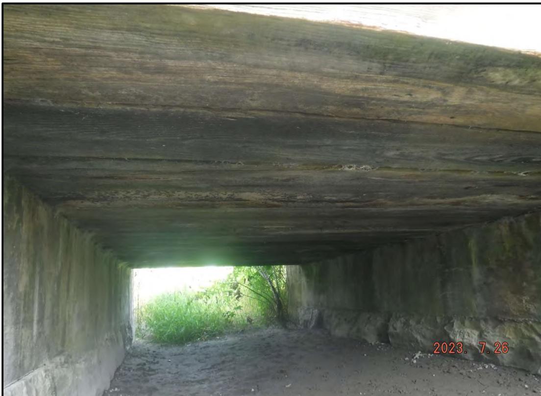
Photo 4: Underside of Timber Slab
