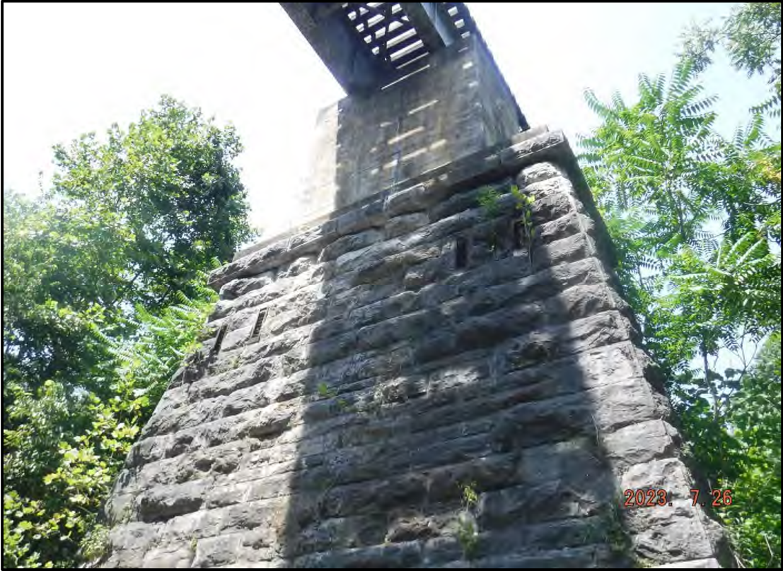
Photo 3: Typical Pier (West Side of Pier 1 Shown)
