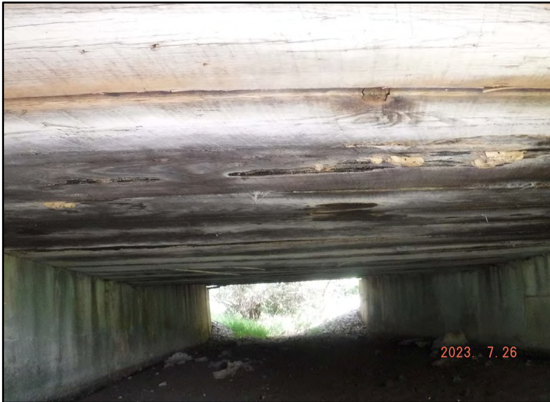
Photo 4: Typical Timber Slab (From North)
