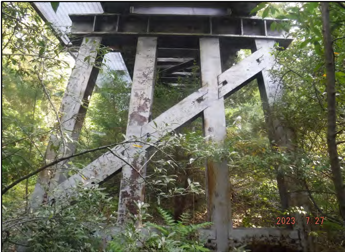
Photo 4: Typical Steel Pile Bent (Typical for Approach Spans)
