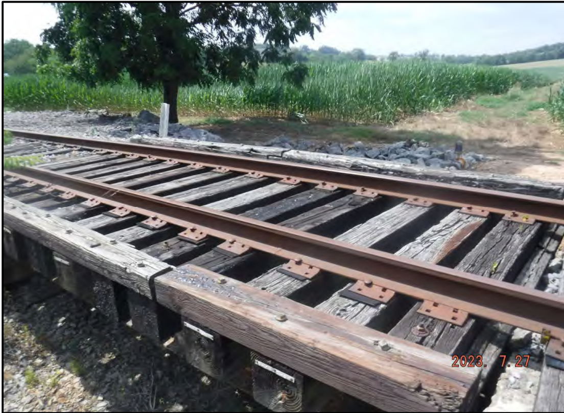
Photo 1: General Condition of Timber Tie Deck
