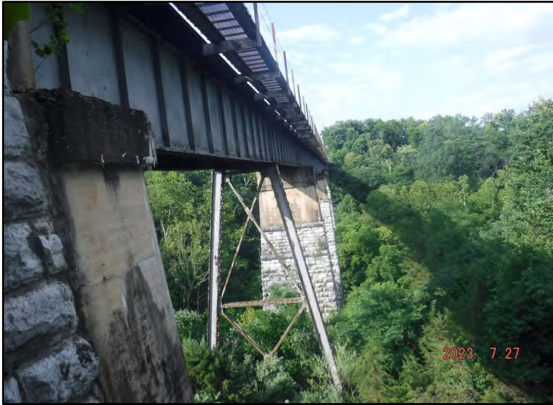
Photo 5: North Side of Main Spans (From East)
