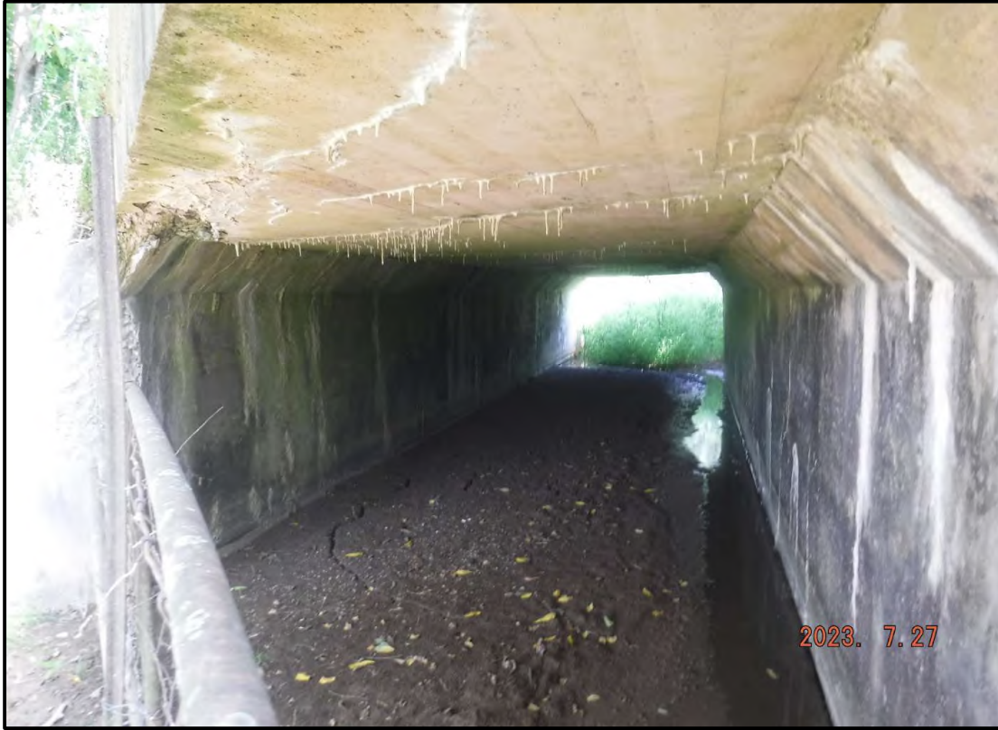
Photo 3: Through Culvert (From North)
