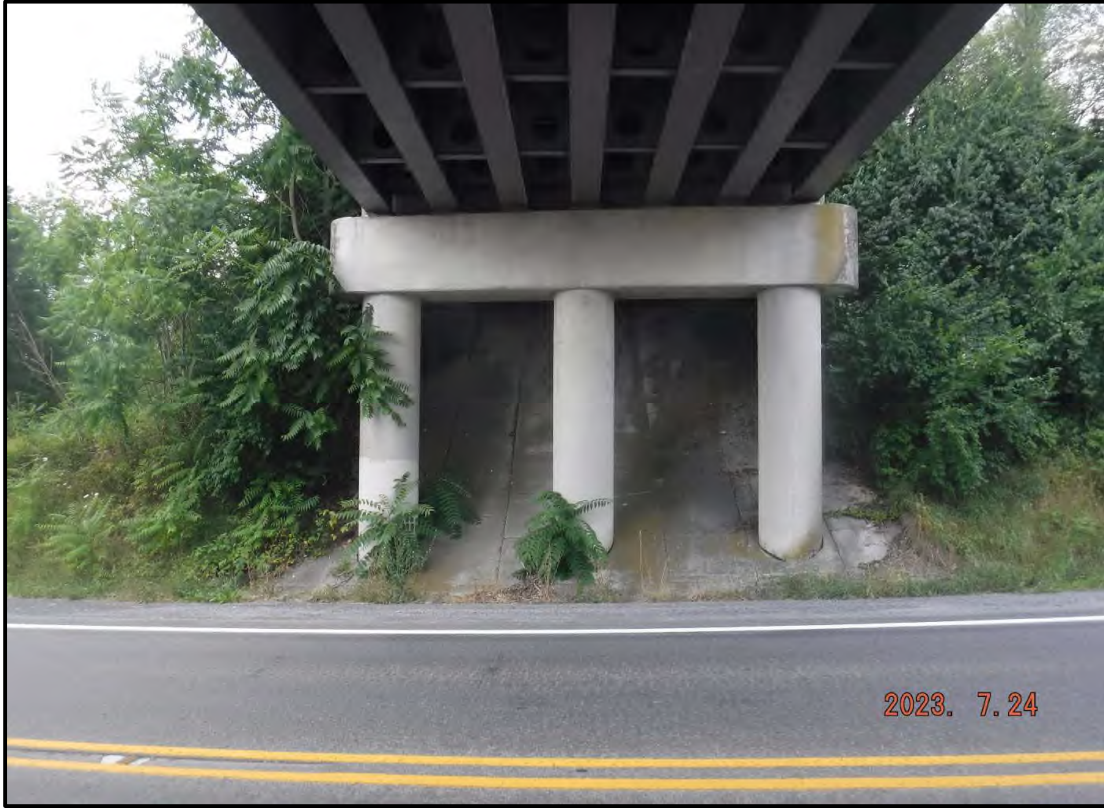
Photo 5: Typical Pier (East Side of Pier 2 Shown)
