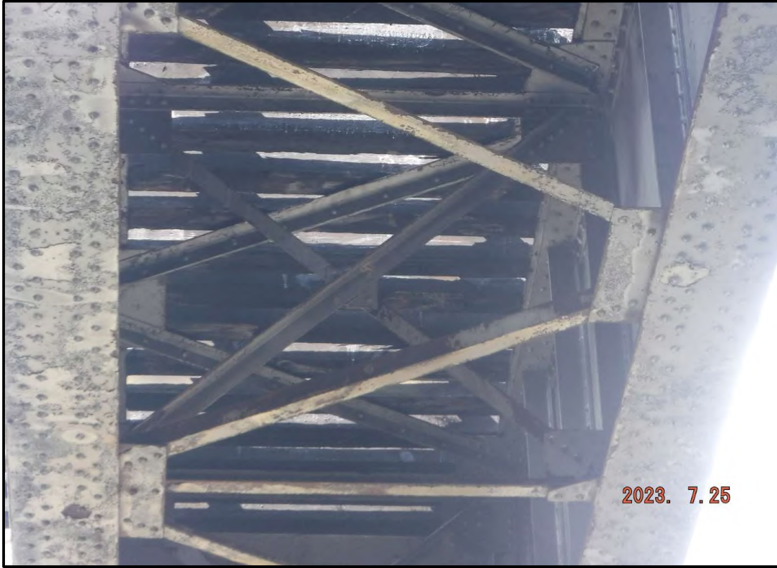
Photo 5: Typical Underside of Span
